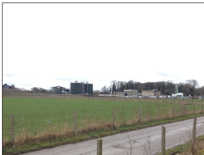
Photo 2:5 View north west from access road towards Five Fords WwTW
