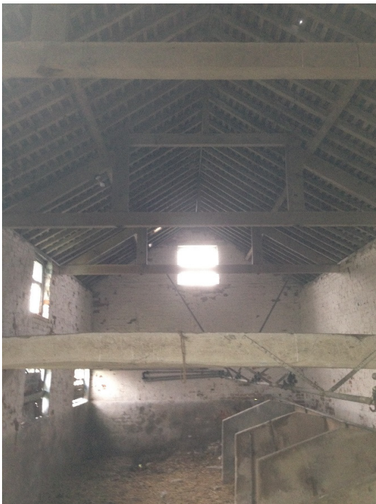
Photograph 11: Truss detail over void in north section of building.
