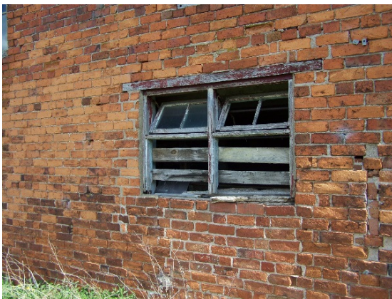
Photograph 19: Later window under timber lintel
