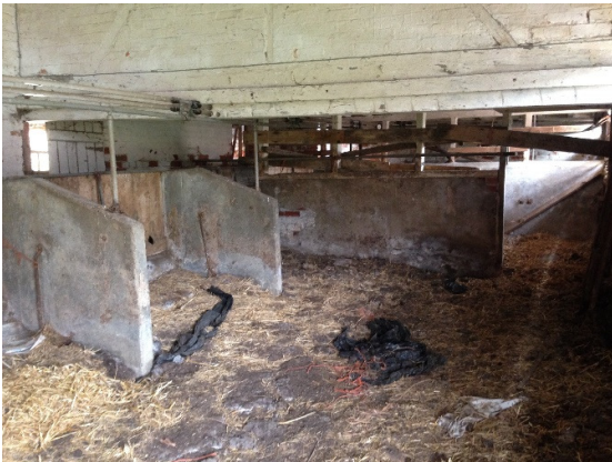
Photograph 13: Cattle stalls in northern section of building. To be removed.
