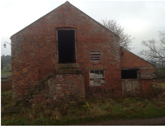
Photograph 1: South elevation of barn, looking north.
