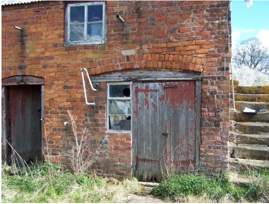
Photograph 9: Brick detail located on the north side of the west elevation.
