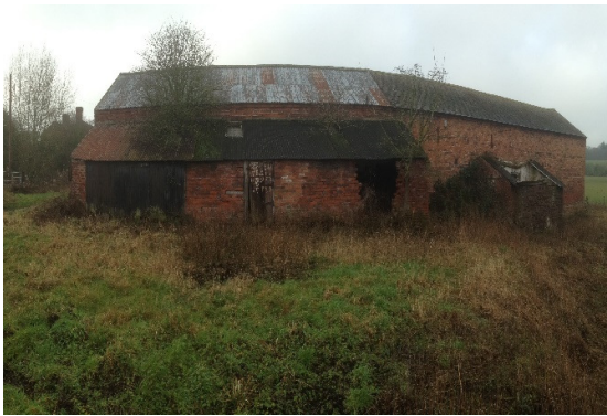
Photograph 2: East elevation of barn, showing lean-to. Looking west.
