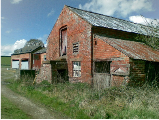
Photograph 15: East lean-to to be retained
