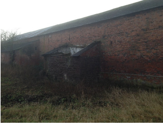
Photograph 4: Lean-to on the centre of the east side, to be demolished.
