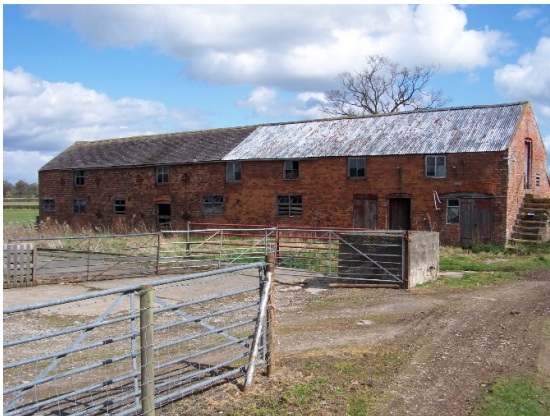
Photograph 3: West elevation of barn, looking east.
