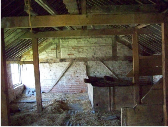
Photograph 12: Queen Post Truss detail on the first floor, south section of building.
