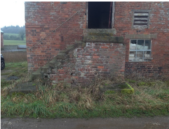
Photograph 5: Staircase on the south elevation.
