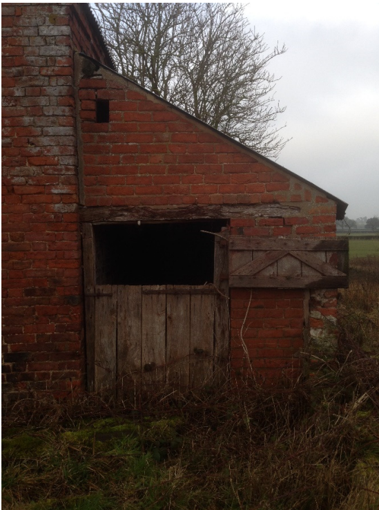
Photograph 6: Doorway on southern lean-to.
