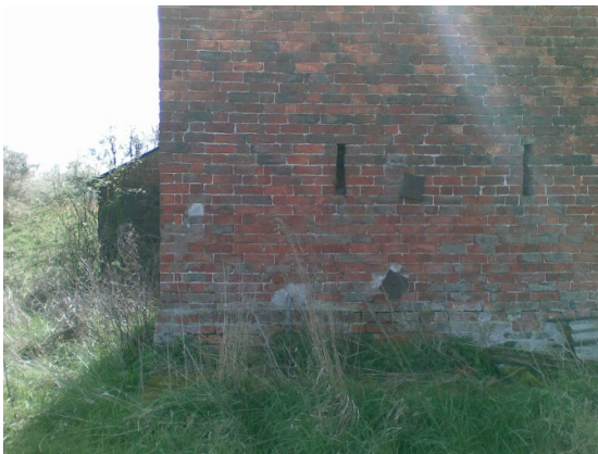
Photograph 10: Brick detail located on the north elevation.
