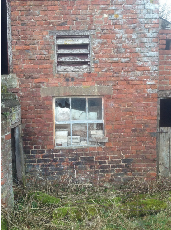
Photograph 7: Ground floor window and first floor air vent on south elevation.
