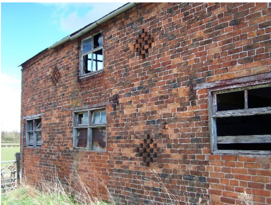
Photograph 17: Evidence of former openings bricked up
