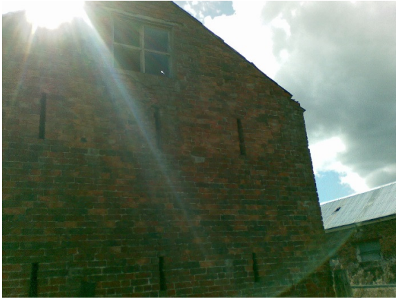
Photograph 21: North elevation window and ventilation slot detail
