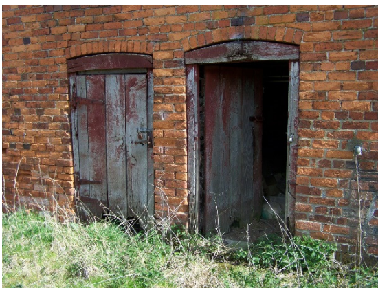
Photograph 20: Simple arched heads to openings
