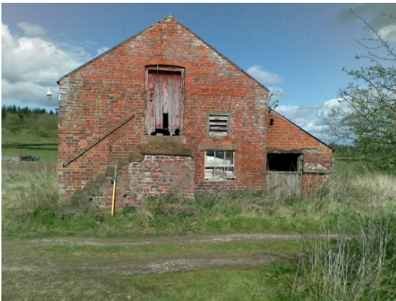
Photograph 16: Granary steps to south side
