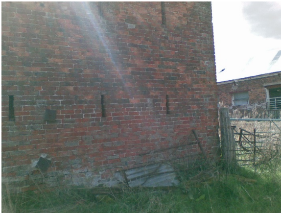
Photograph 22: North elevation window and ventilation slot detail
