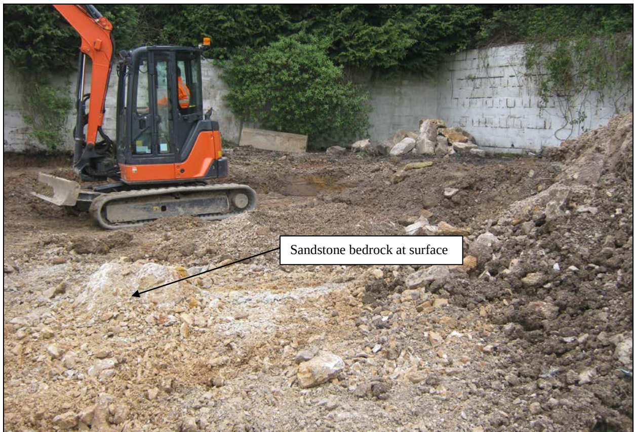
Figure 11: Photo from the eastern boundary showing rockhead at surface
