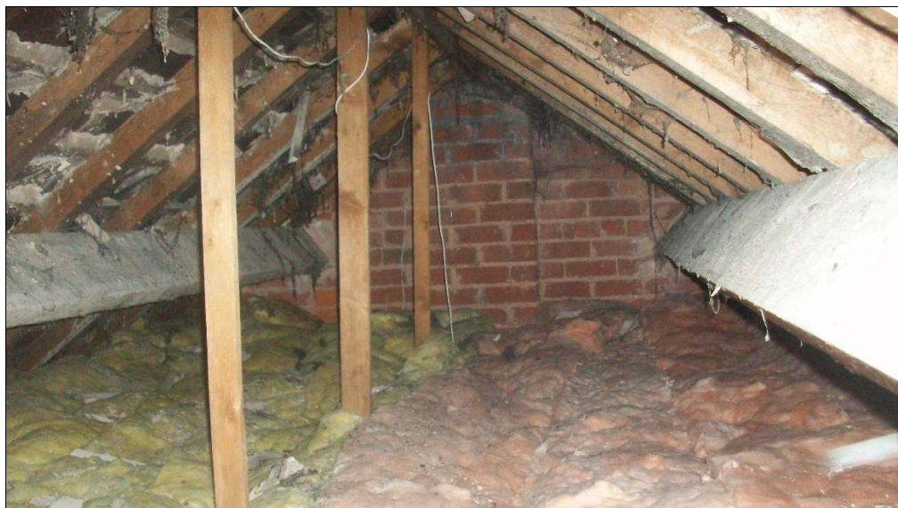
Plate 6 – The roof void within B1a, note the extensive amount of cobwebs
