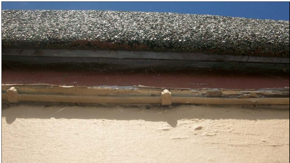
Plate 4 – Showing the fascia boards of B1b. No gaps present.
