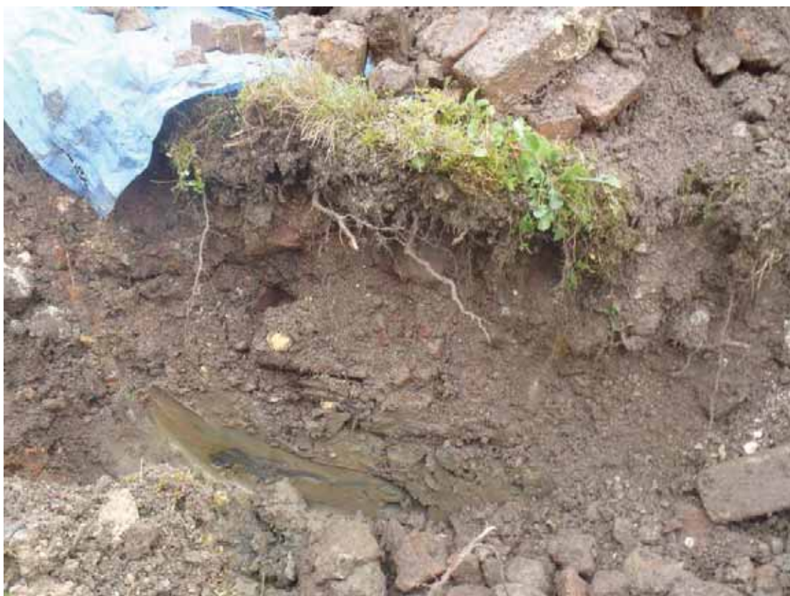
TP24: Showing 0.6 m sandy Made Ground with brick and concrete fragments overlying silt (alluvium)
