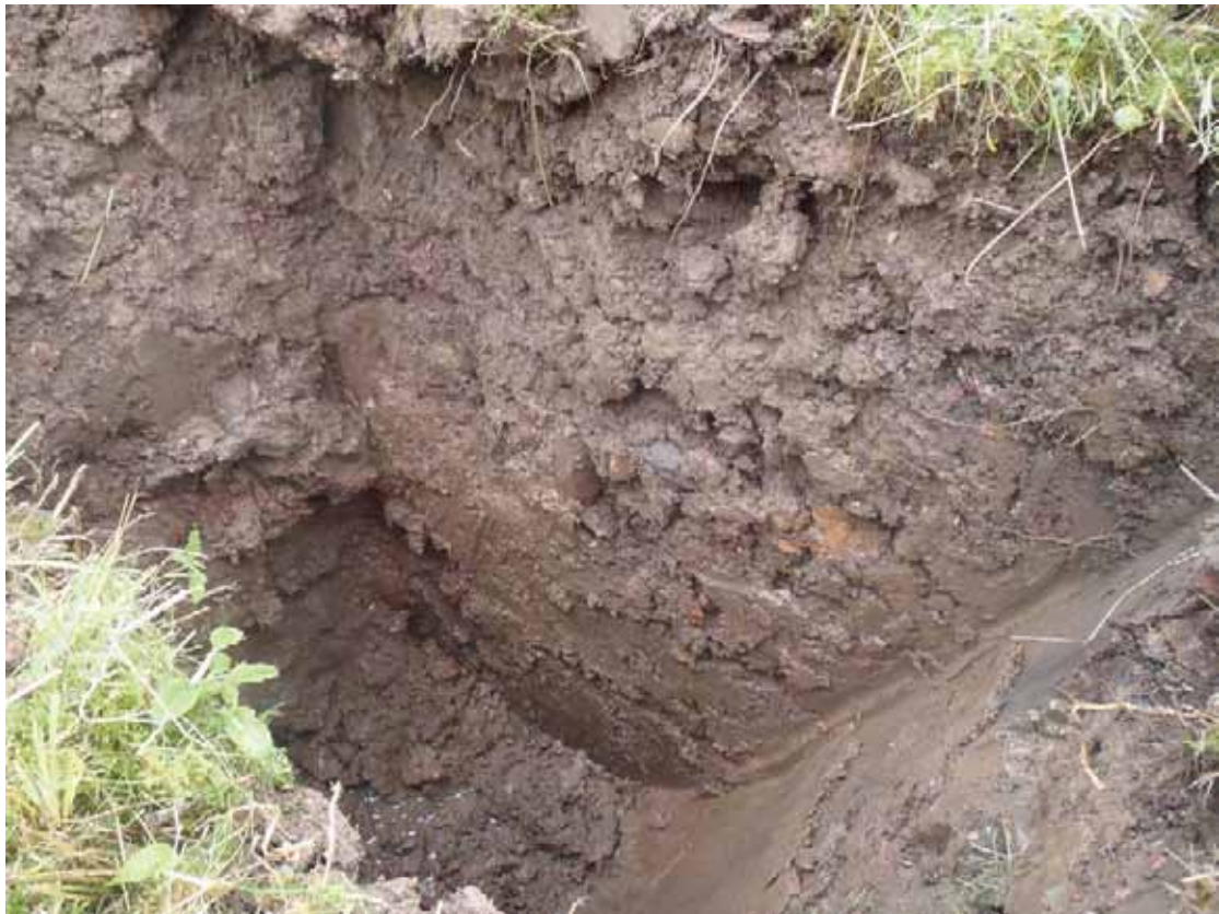
TP16: Showing Made Ground to base of trial pit (1.4 m) with minor seepage evident
