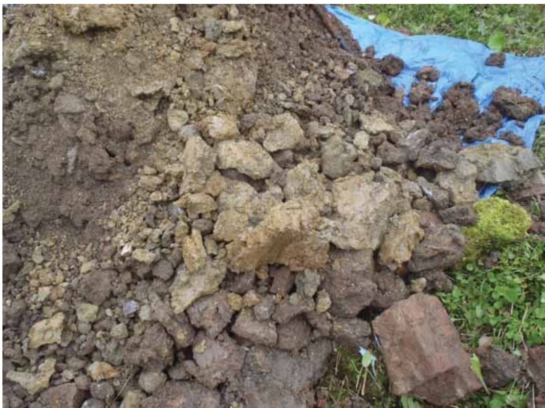
TP3: Showing silt (alluvium) found at base of trial pit
