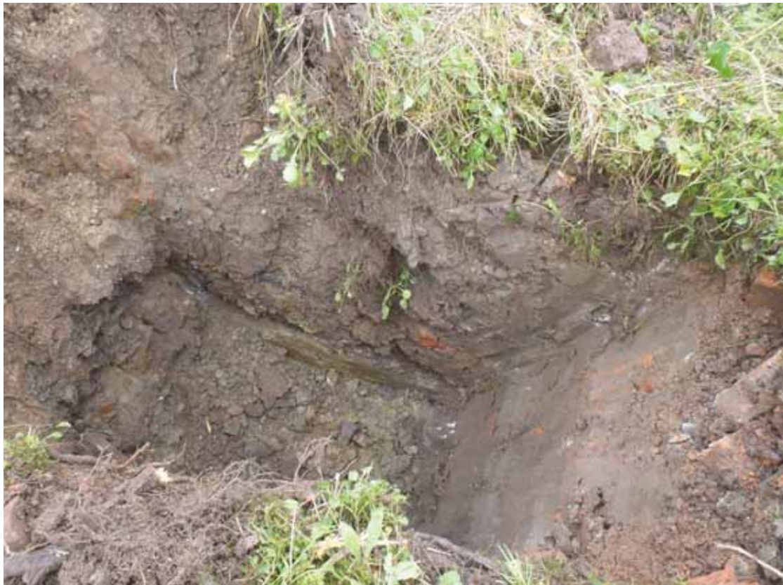
TP3: General view of trial pit showing alluvium at base
