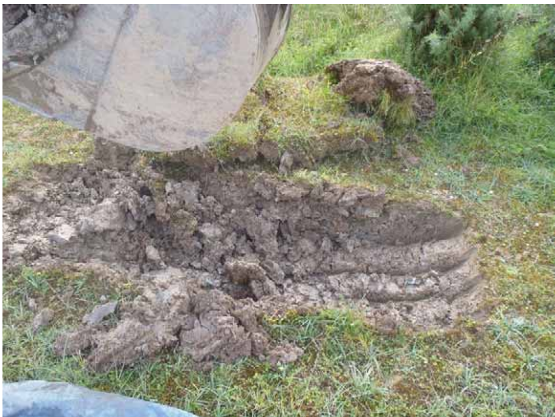
TP10: Showing glacial till below 0.2 m of clayey Made Ground
