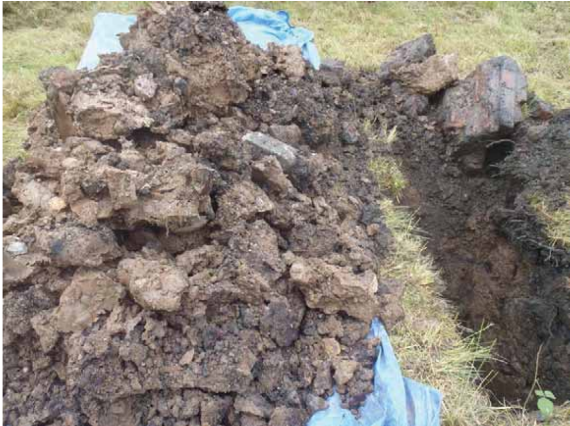
TP22: Showing general view of Made Ground from trial pit
