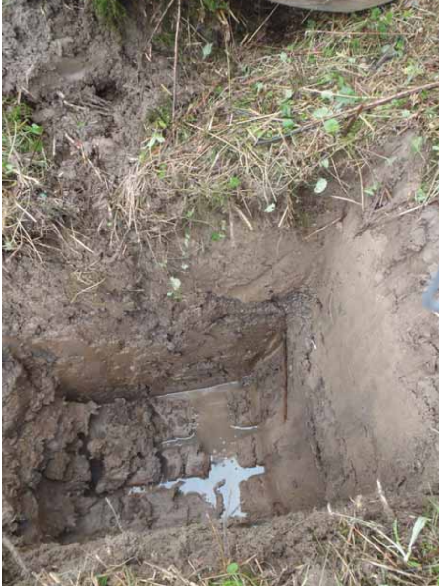
TP32: Showing 1 m layer of clayey sandy Made Ground above soft clay (glacial till). Water strike at 0.5 m within Made Ground
