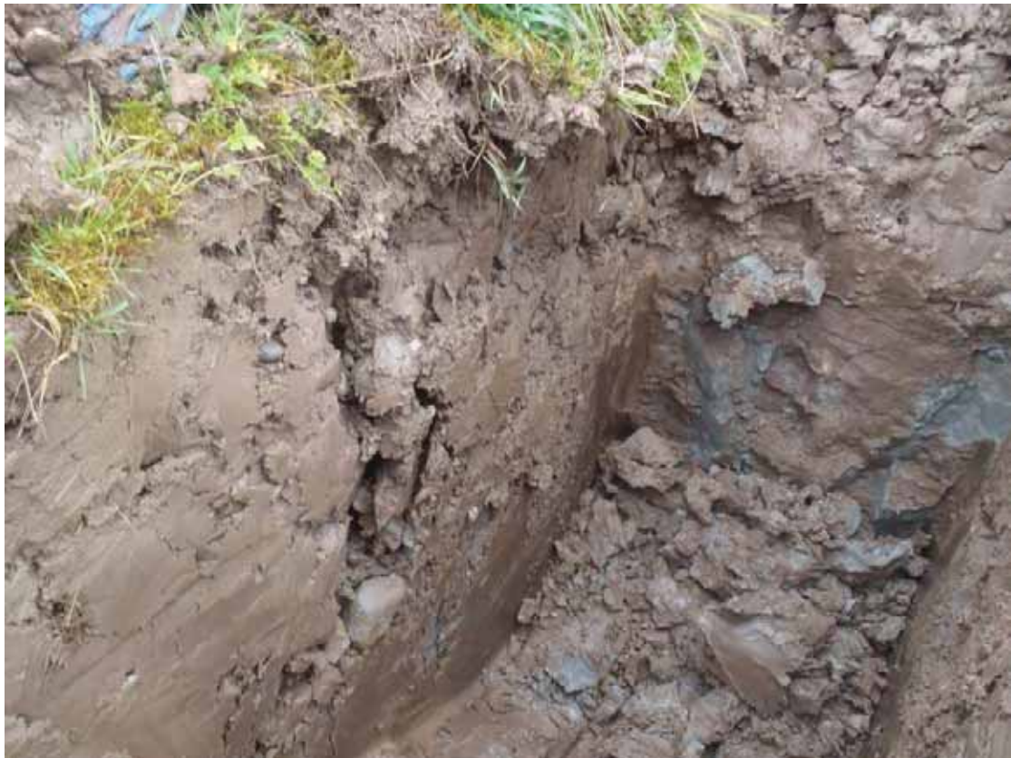
TP31: Showing 0.5 m layer of clayey Made Ground with occasional tile / brick fragments above stiff clay (glacial till)
