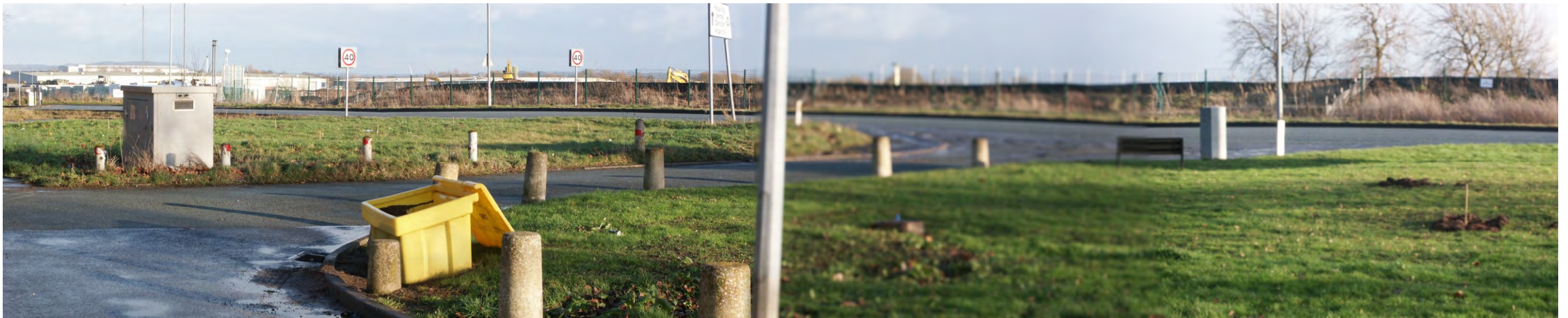
Plate 23 – Photograph taken road adjacent to housing at Pentre Maelor within the existing Industrial Estate looking south west towards the proposed site with the Prison Site under construction in the foreground
