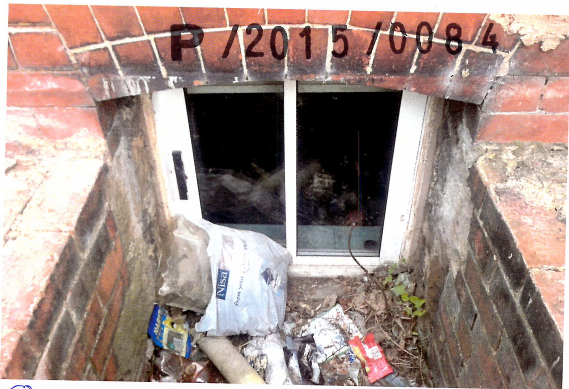
① cellar window - old.
