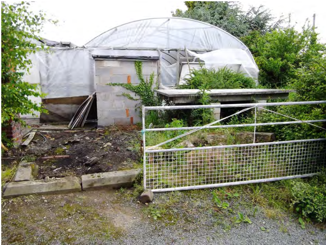
Photograph 5 former oil tank locations near entrance
