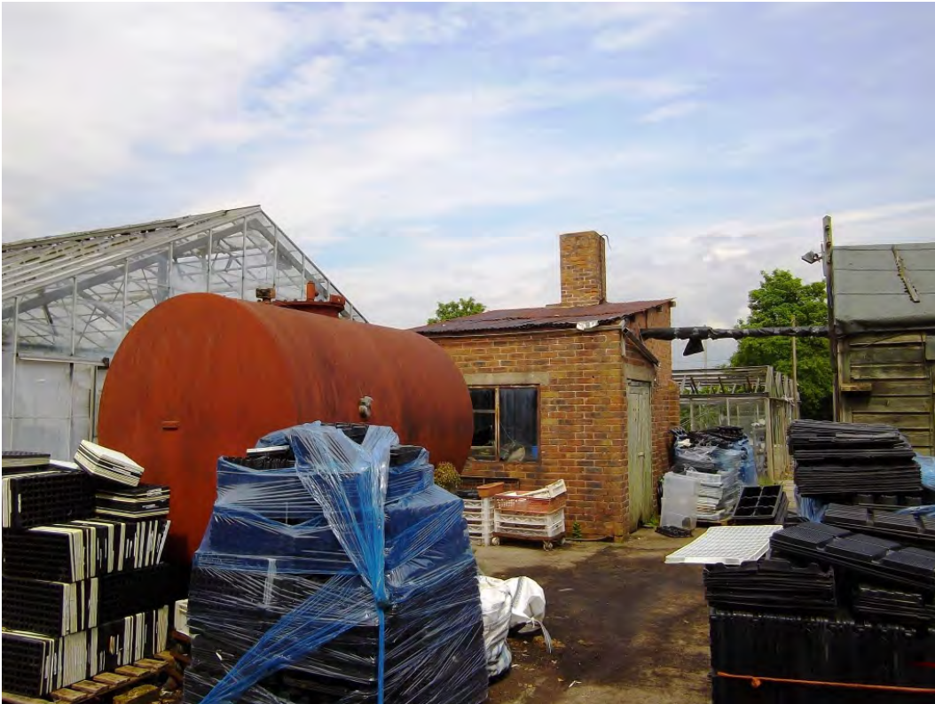
Photograph 19 Oil tank and boiler in central section of site
