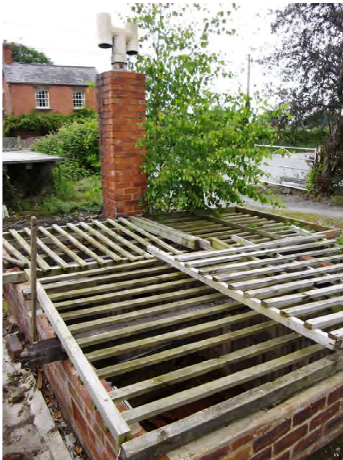
Photograph 6 Location of former underground boiler
