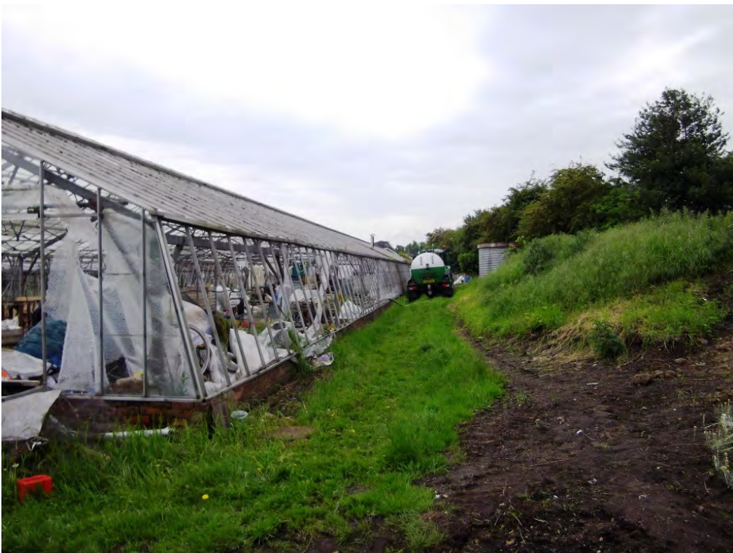
Photograph 14 Looking south from NW corner
