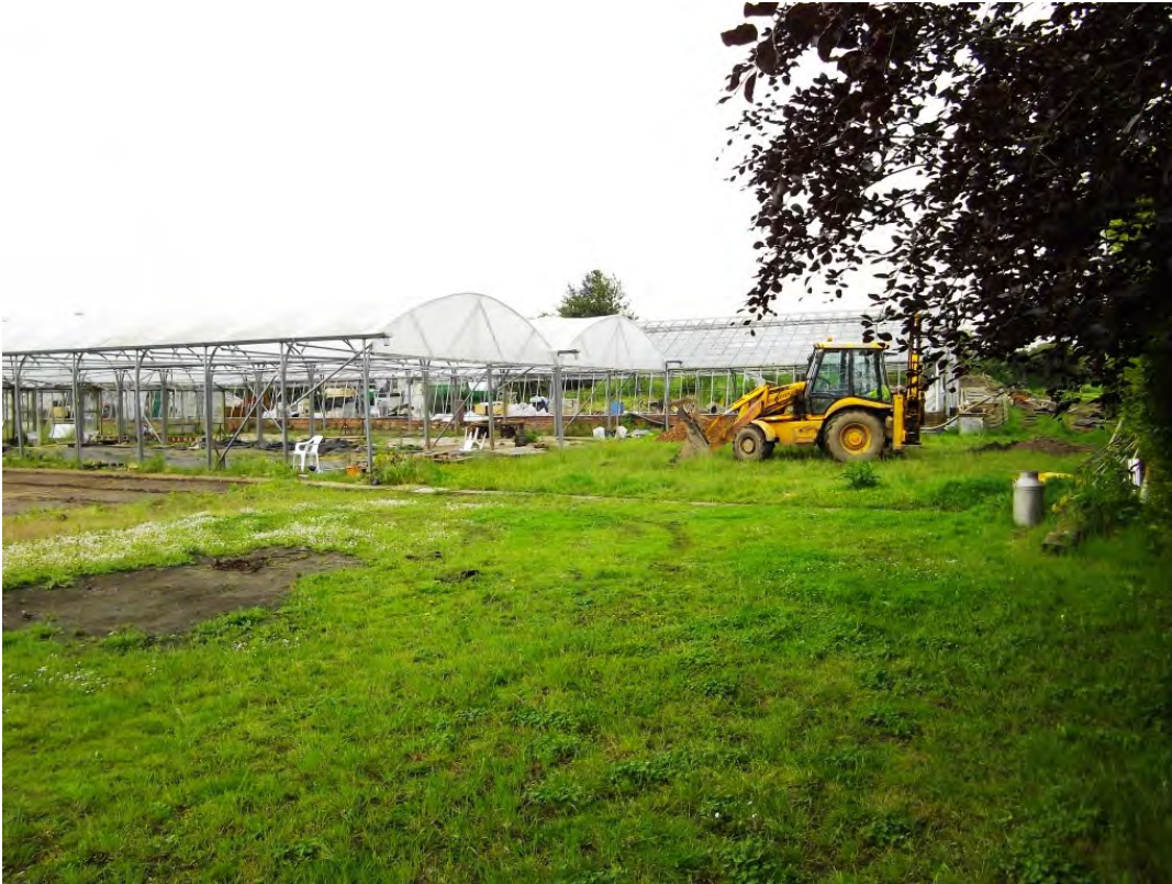
Photograph 17 Looking west from NE corner
