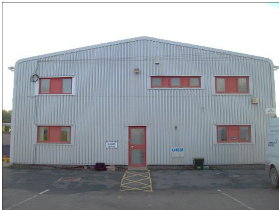
Figure 4: A view of the front of B1 from an eastern viewpoint.
