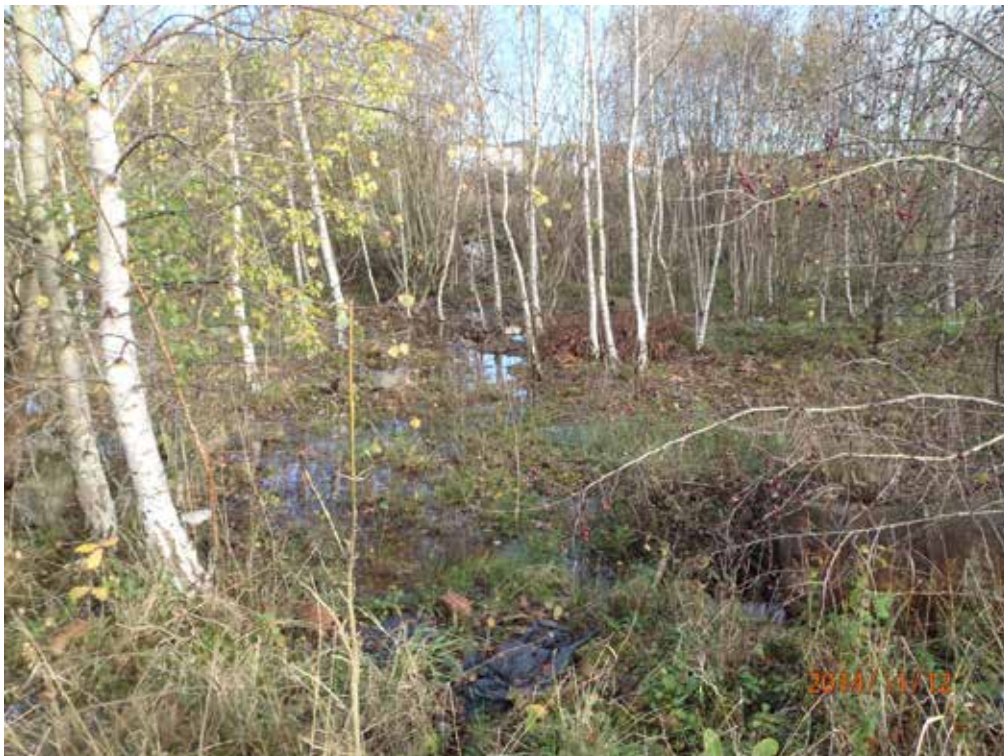
Plate 2: View of the broken concrete pad with associated vegetation and an area of standing water - believed to be wet as a result of a recent burst water pipe
