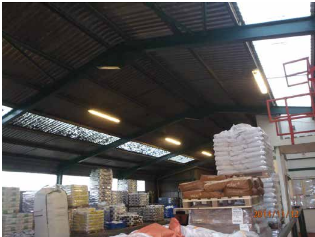
Plate 10: Internal view of the main building, showing its unsuitability to support roosting bats
