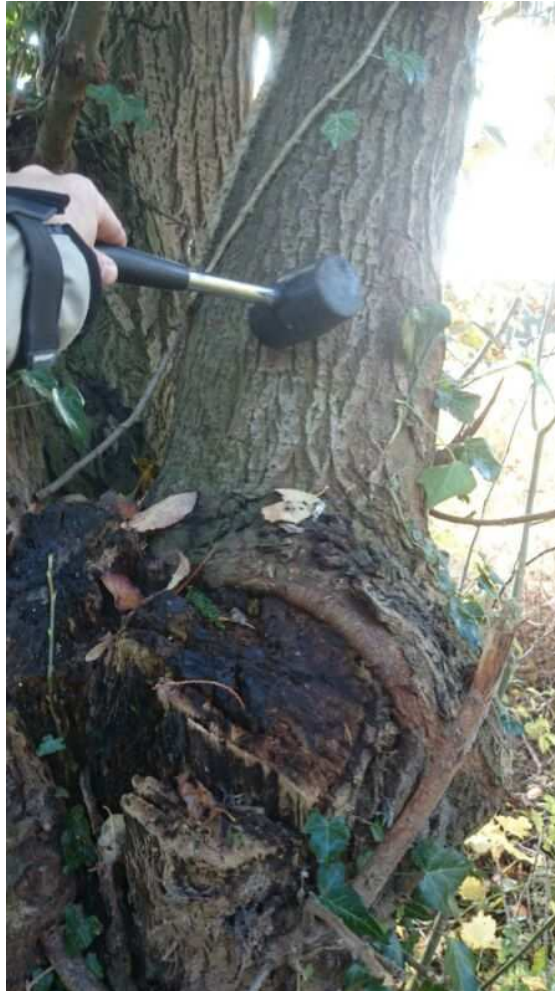
Picture 2 Stem where decay was found on 521
