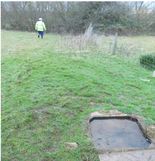
Plate 2: Blocked drain leading to outfall to ox-bow lake located North of SS11-06-1 (10-12-2014).
