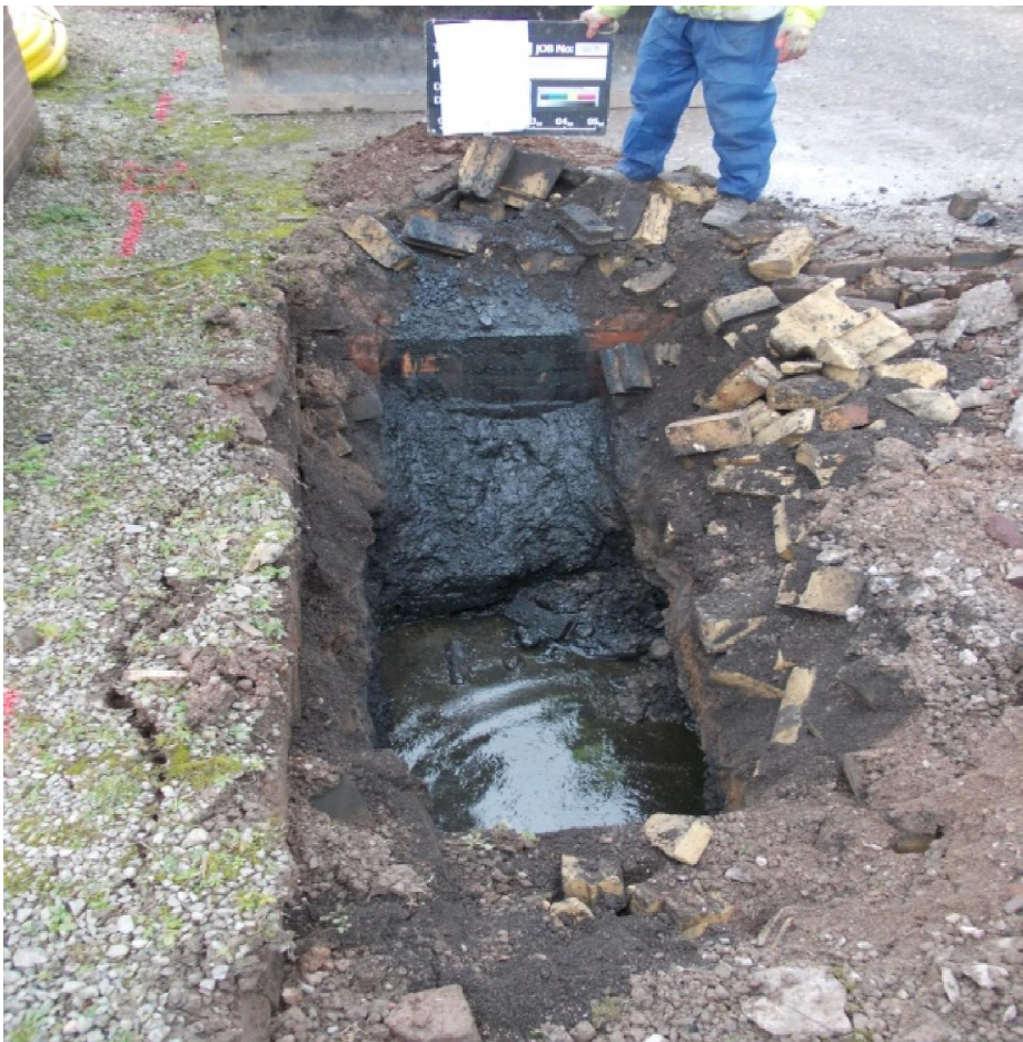
Plate 10: TP1 South of Garage (29-11-2013)
