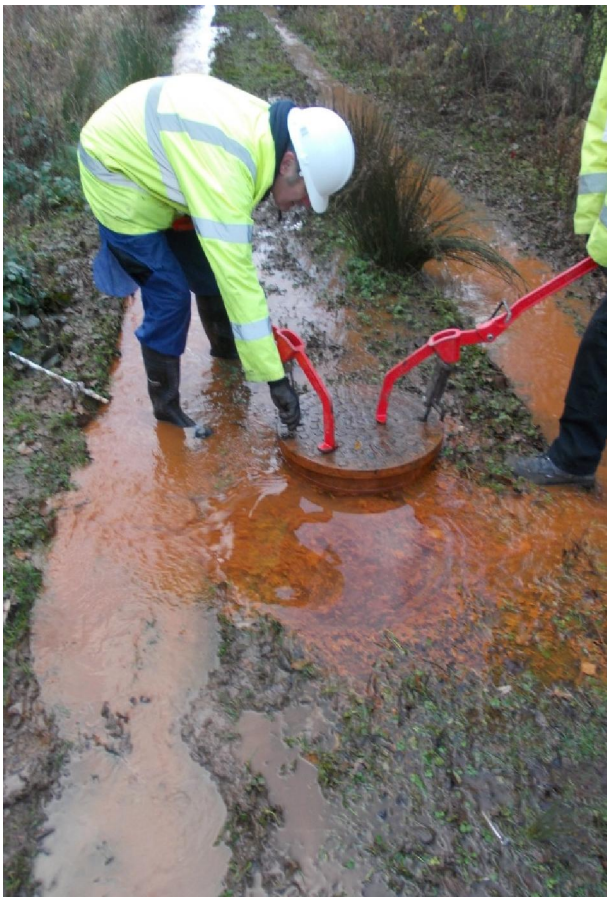
Plate 6: Leaking Water Main on Northern boundary track SS11-05-01 (10-12-2014).
