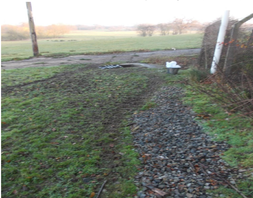
Plate 4: French Drain (SS11-07-1) NW Boundary – Looking North (10-12-2014).
