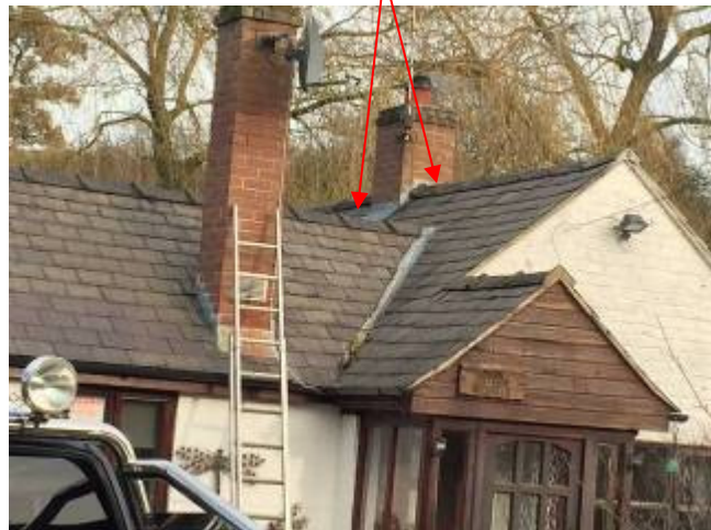
South, east & north elevations of Moor cottage – two raised ridge tiles either side of chimney breast
