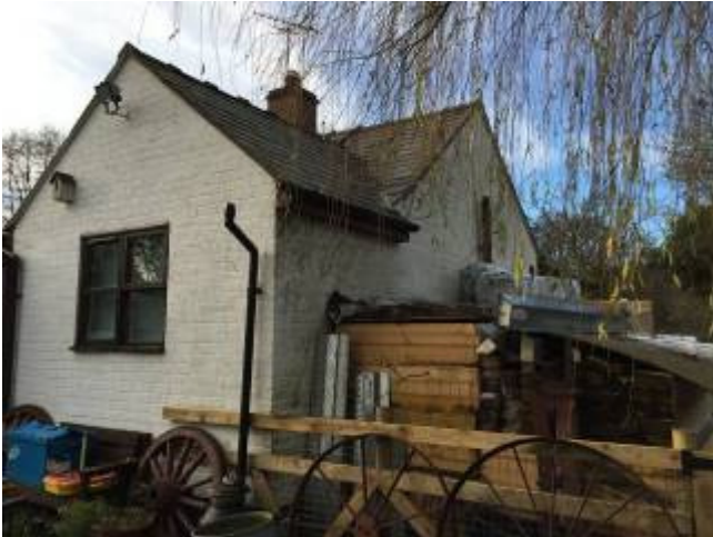
South, east & north elevations of Moor cottage – two raised ridge tiles either side of chimney breast
