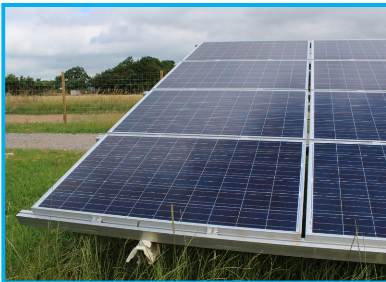
Fig 10 Typical solar array showing 20mm thermal gaps between panels to disperse runoff.
