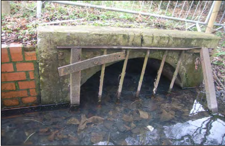
Plate 9 – Close up of culvert outfall
