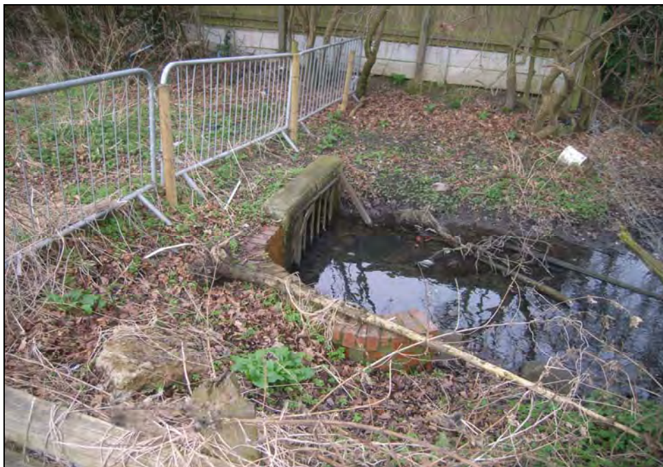
Plate 8 – Culvert outfall.
