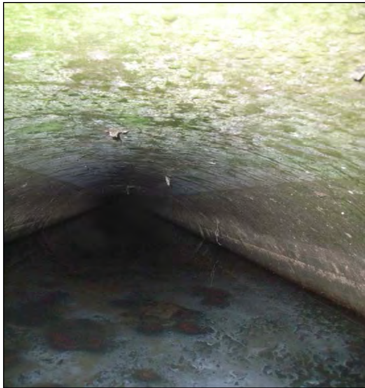
Plate 10 – Looking south down the culvert
