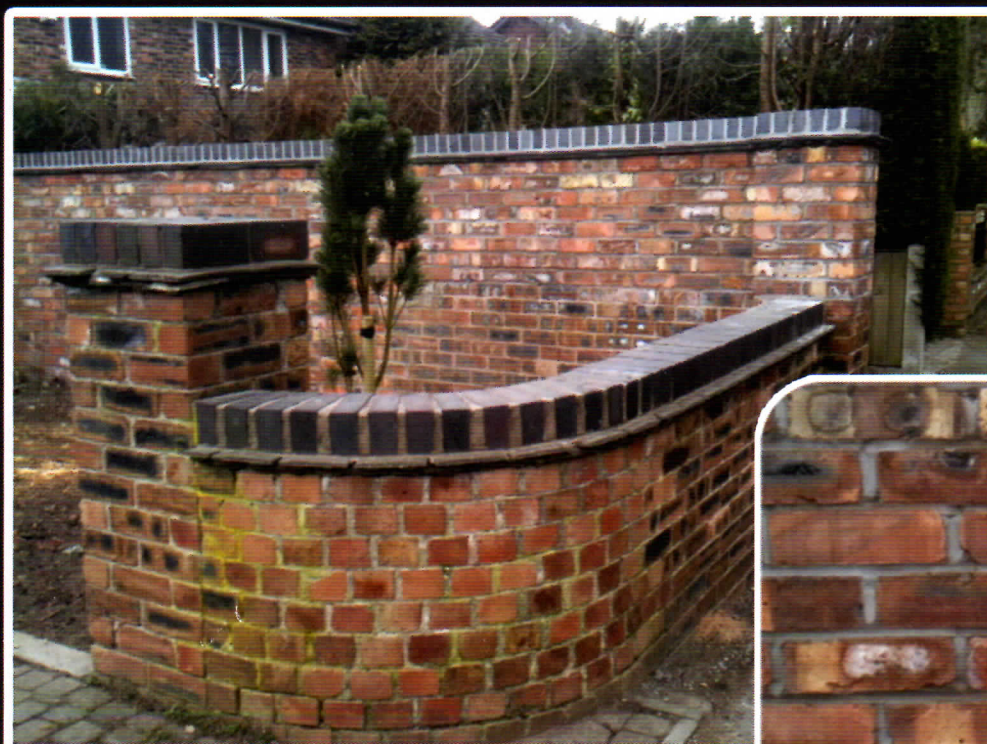
The above shows an extension to a wall using the new scotch common against the old original caradale scotch common.
