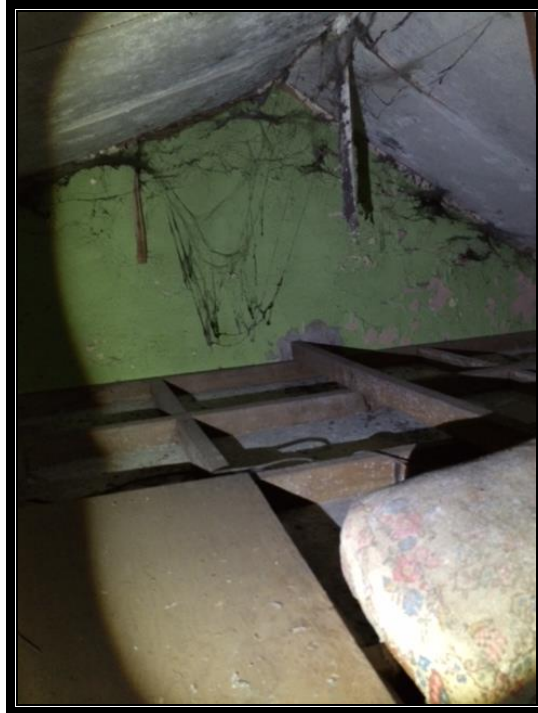
Building 2; loft void.
