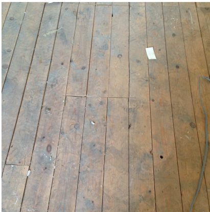
The floorboards proposed to be lifted to form the new stairwell are modern T&G
