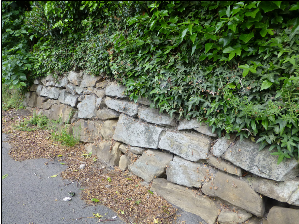
Photograph 4: The bank is partially retained by a dry-stone wall
