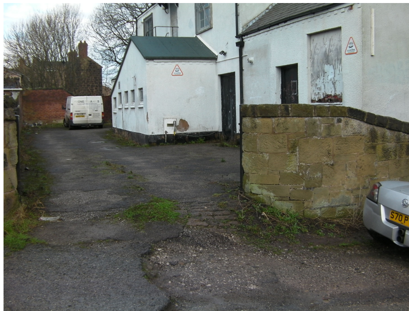
Fig. 1 Existing Access Point
