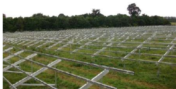
Frame structures prior to attachment of panels
