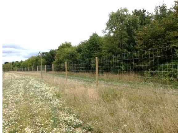
Fence at Tavells Solar Farm, Hampshire
