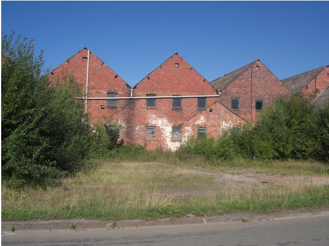
Part B Front showing area of Demolition
