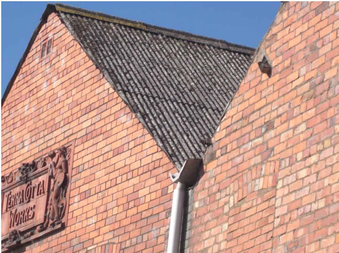
Typical Roof Tiling / Internal Gutter
