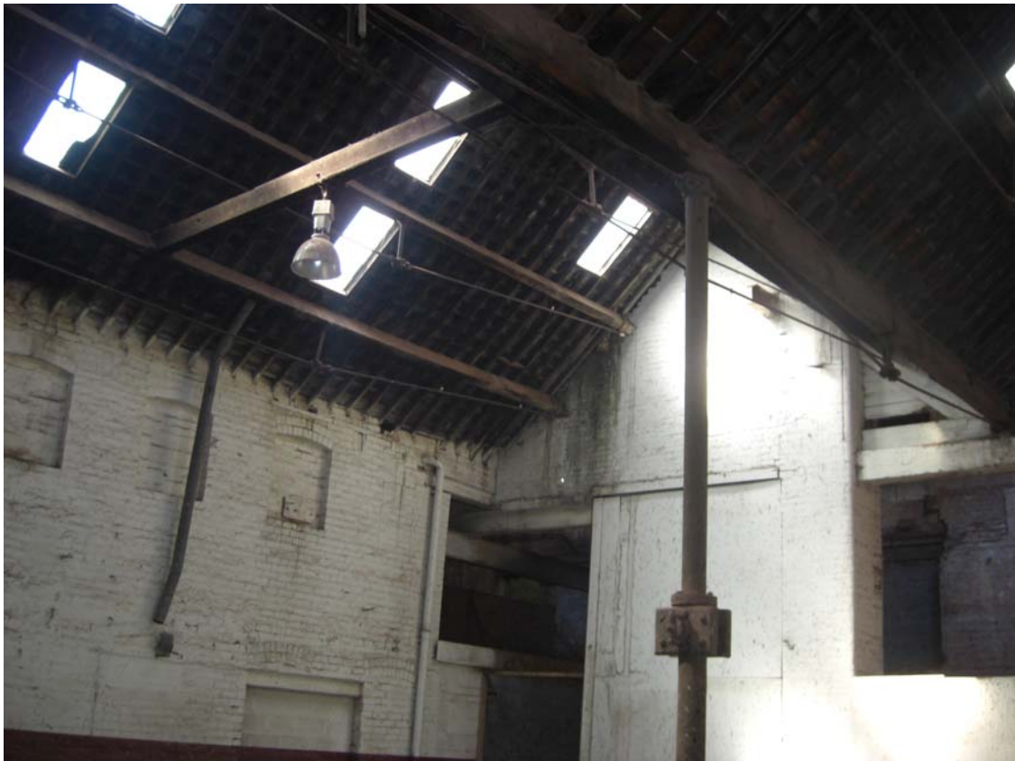
Typical Internal Part B - With roof prop
