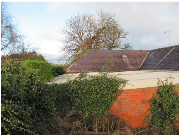
Single storey brick extension to the rear of the original Smithy building
