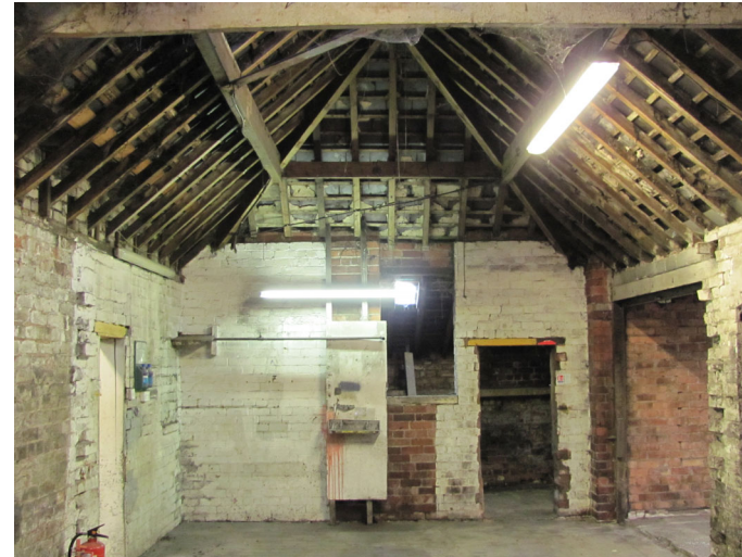
A view of the early outrigger to the extended Smithy building before it became a tyre depot
