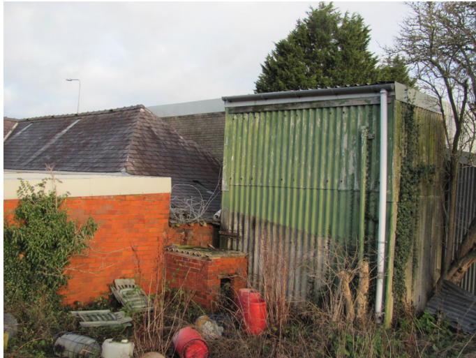
The rear of the tyre depot and the steel clad storage buildings
