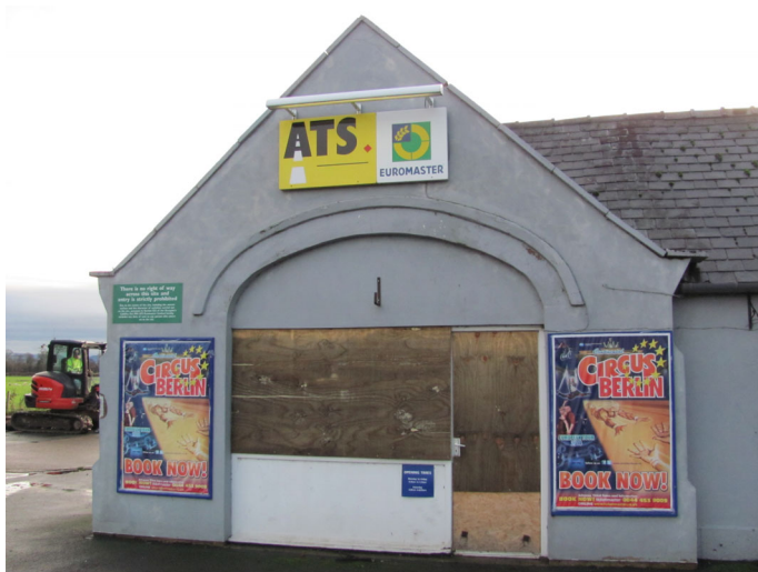
The later addition of a wider gable to create some symmetry to the building's front elevation
