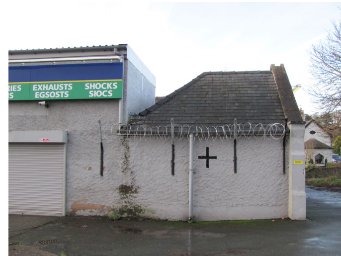
View of the north eastern elevation and the additional extension probably built in the late 1950's
