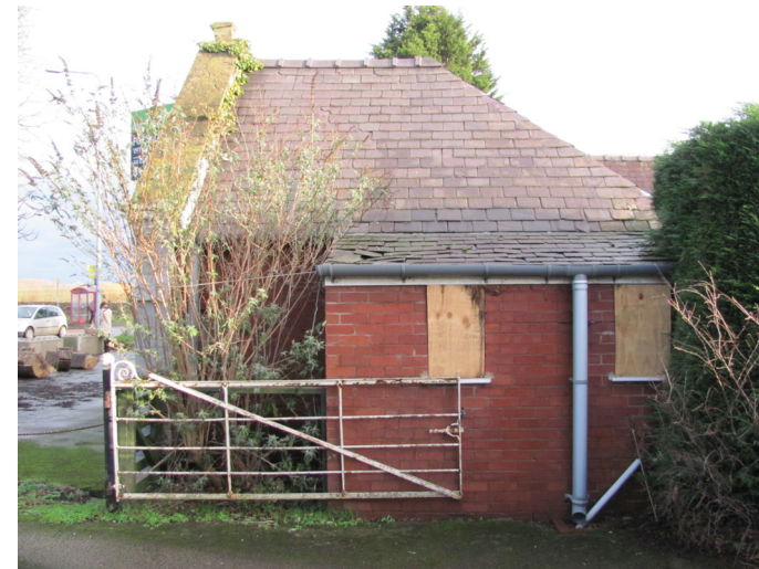
The south western elevation that faces Smithy House. The toilet block which is to be removed to provide a secure maintenance strip
