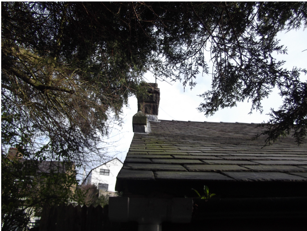
Picture 7 Para-pit wall above roof line.
