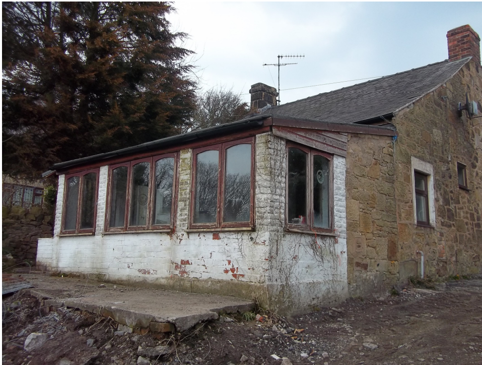
Picture 11 Extent of conservatory
