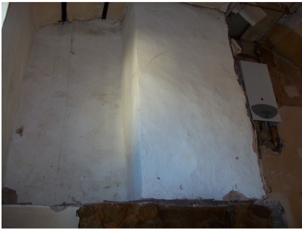
Picture 15 Chimney breast first floor
