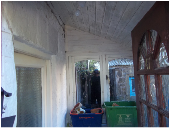
Picture 13 Front entrance porch
