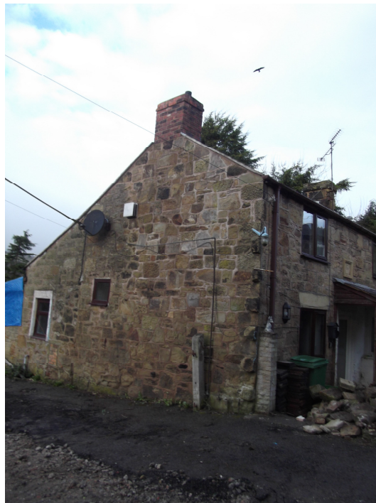
Picture 3 Side elevation with continua's roof slope
