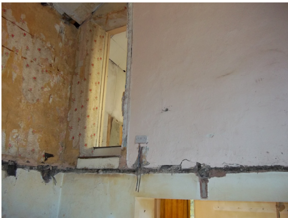
Picture 17 First floor bedroom entrance
