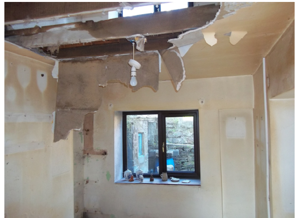
Picture 16 Ground floor window
