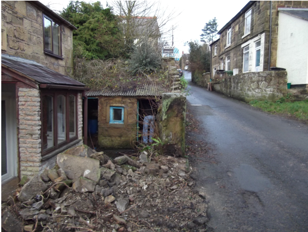
Picture 2 Shed to front of property
