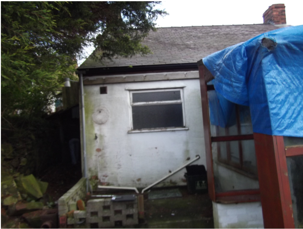
Picture 6 Rear elevation bathroom window
