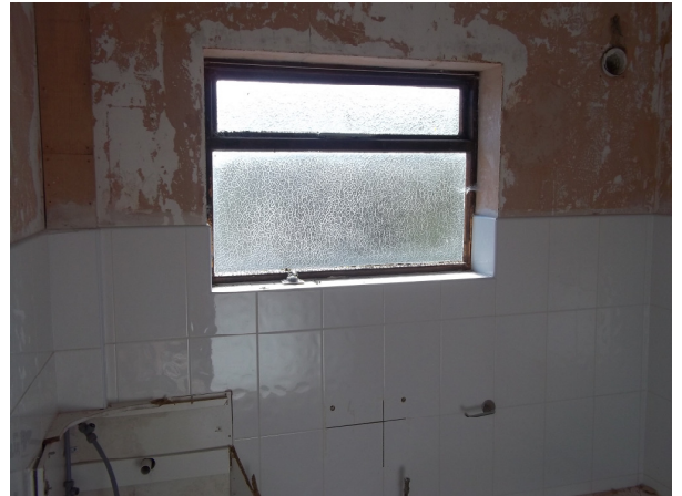
Picture 18 Ground floor bathroom
