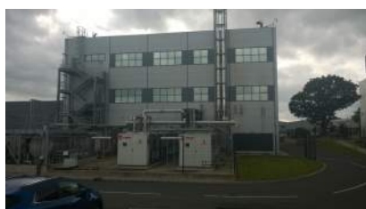
Building 12 with flat cladding
