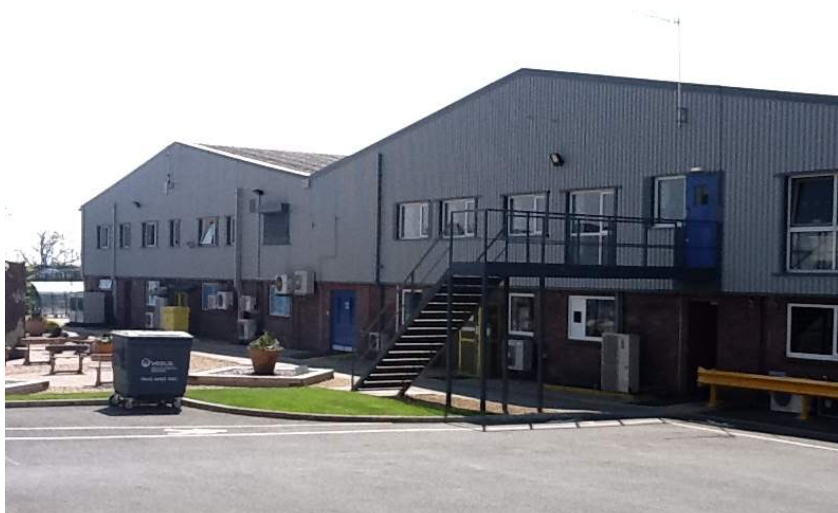
Fig 2. Exterior view of the north face of building 9
