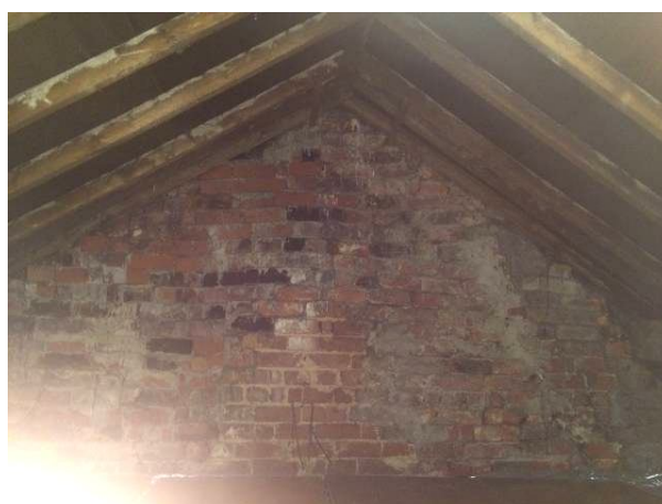
Photo 4: Internal View of roof void.
