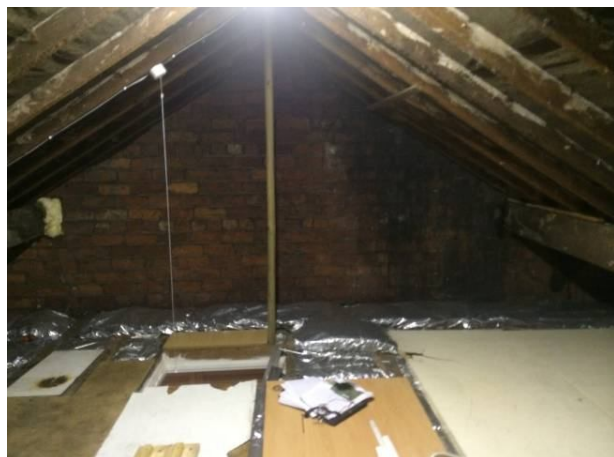
Photo 3: Internal view of roof void.
