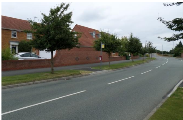
Photograph 3 Bus stop on Croesnewydd Road
