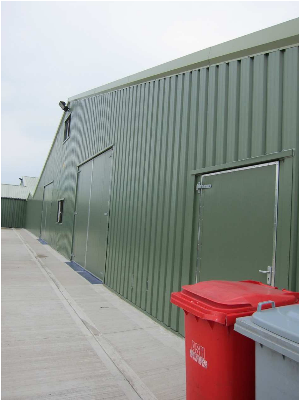
The front of the building – the manure at end of 60 week cycle is taken out through the double doors at end.
