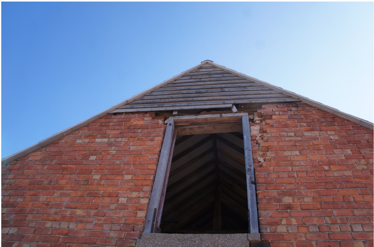
Figure 3: End with weather boarding
