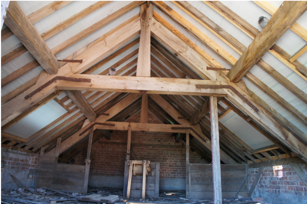
Figure 4: First floor of building
