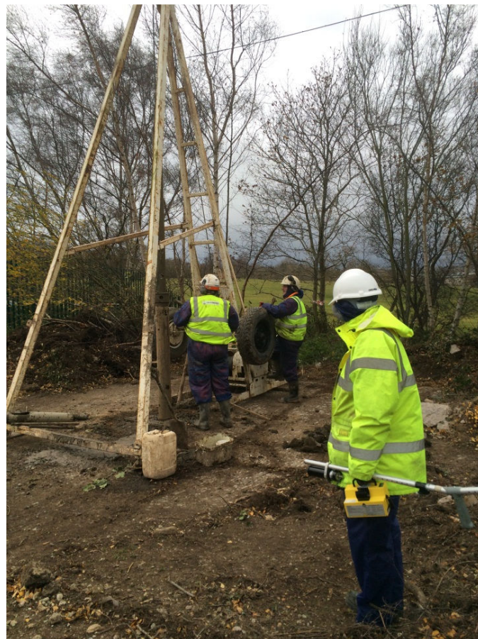
Figure A8 Supervising and monitoring drilling works.
