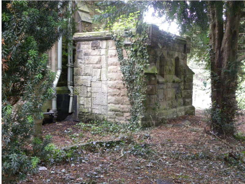
Photograph 3. showing the Cemetery Chapel Toilet (to be demolished).
