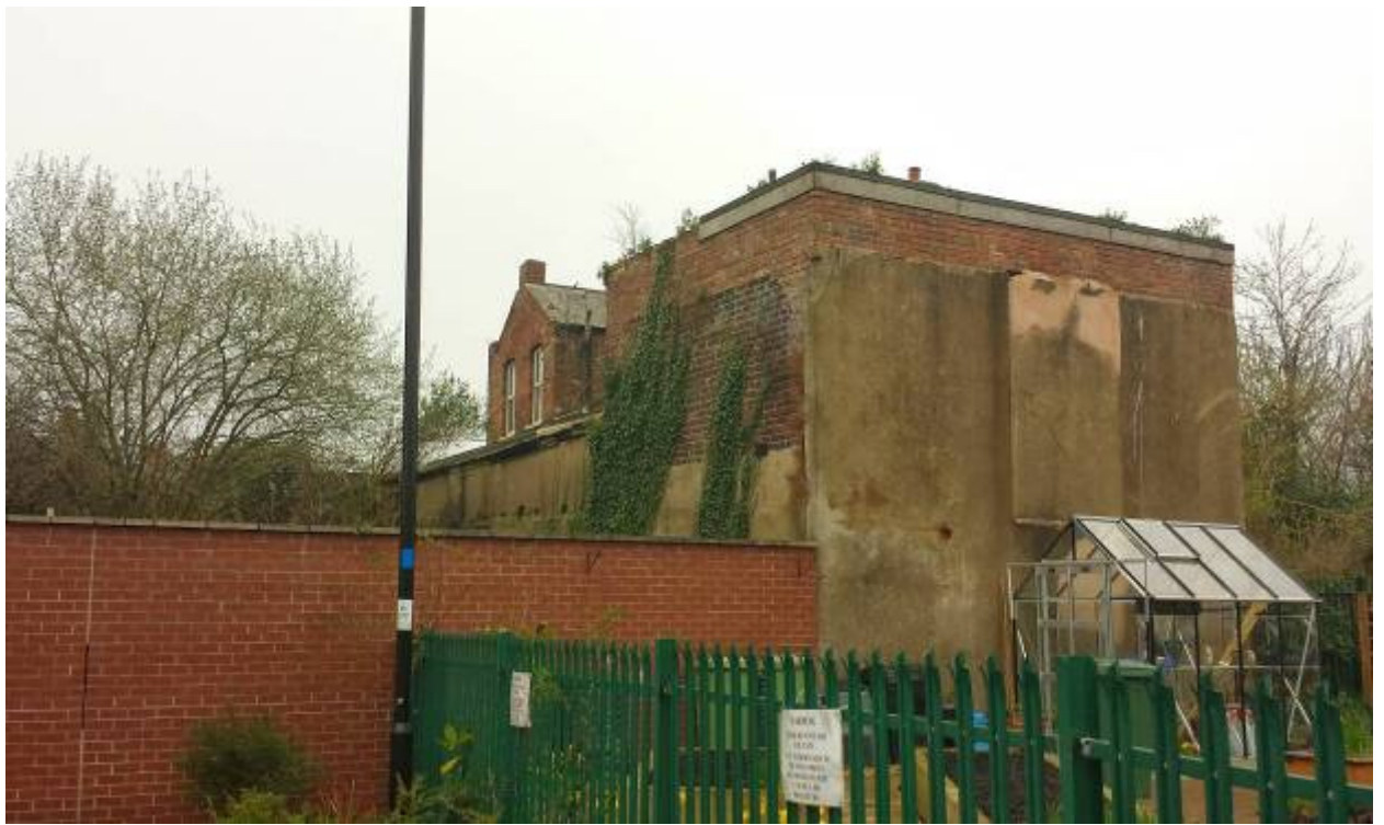
Side elevation of 17 Manley Road
