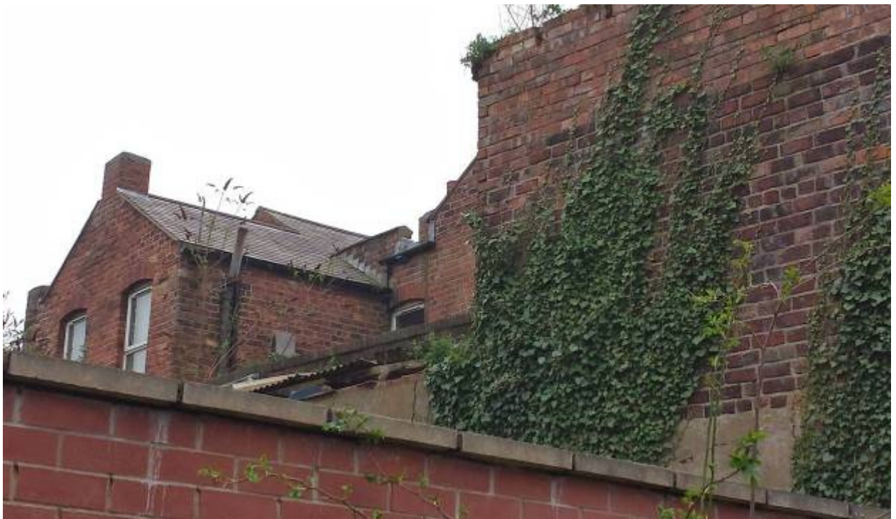
Complicated roof structure with restricted view at 17 Manley Road Wrexham
