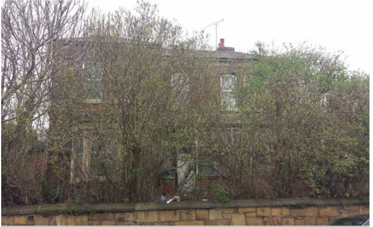
Front elevation of 17 Manley Road
