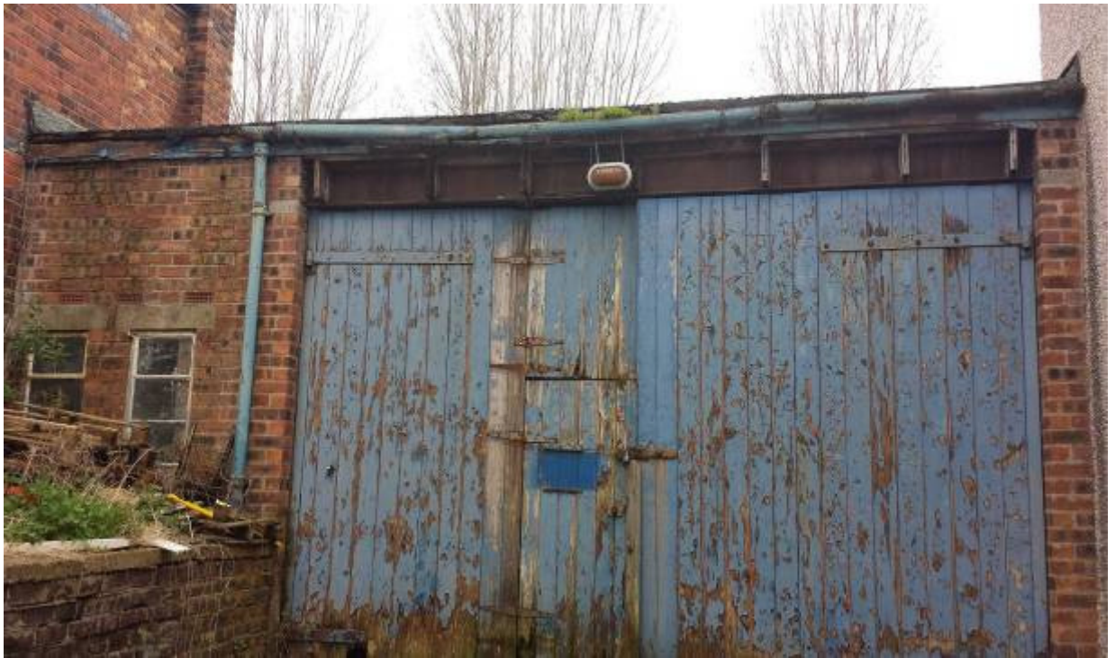
Front of the garage at 17 Manley Road
