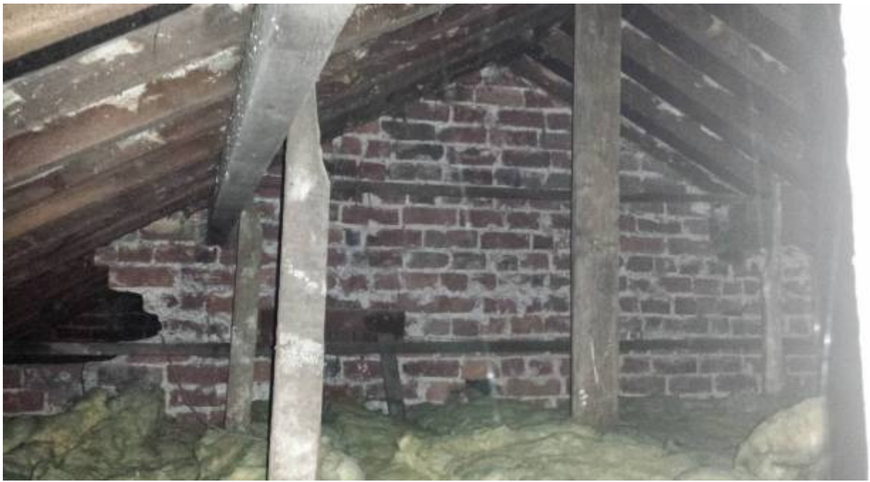
The inspected loft space at 17 Manley Road
