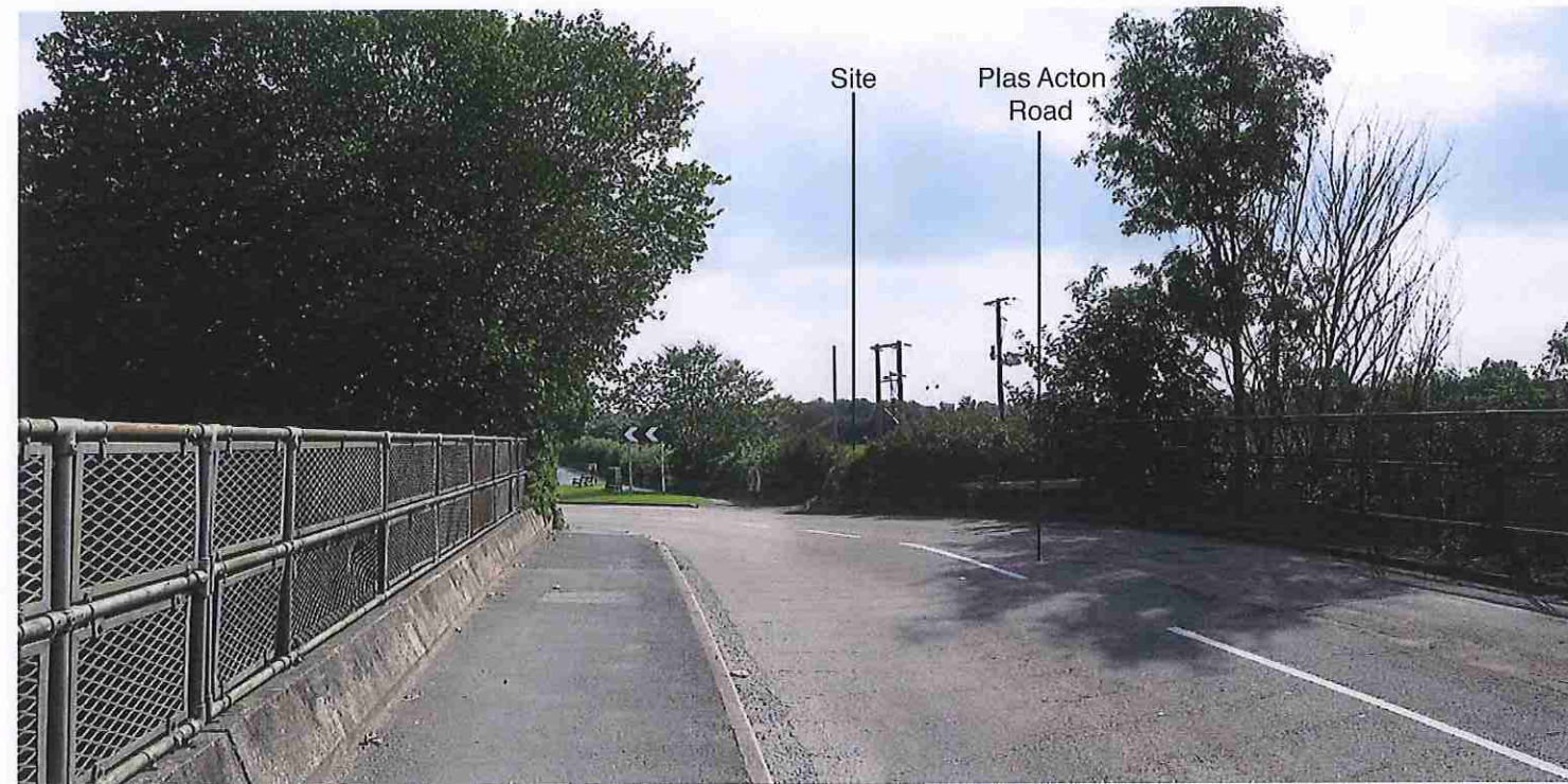
Photograph 12: View from railway bridge along Plas Acton Road towards site
