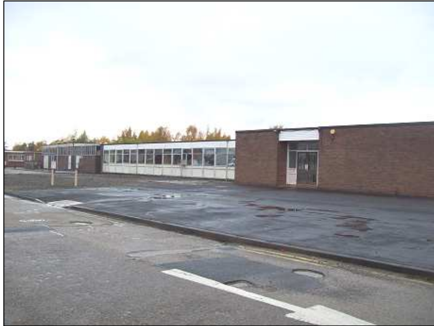
Figure 11: Building 1 (B1) and some of the hard standing from a south-eastern viewpoint.
