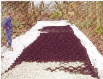
CellWeb during installation.
