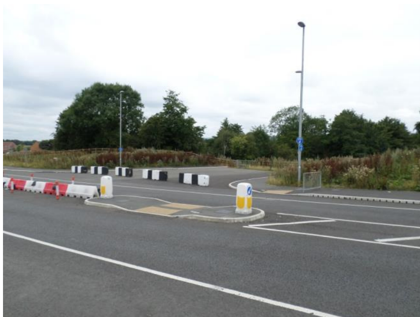
Photograph 1 Junction stub which will provide site access
