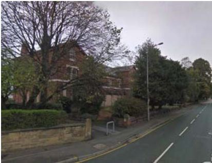
Fig 3. View of existing site from Grosvenor Road
