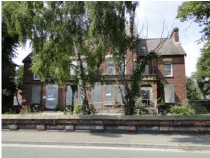
Fig 16. Existing front boundary wall
