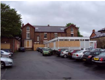
Fig 5. Rear of Block 1 along with previous Hostel Extension.
