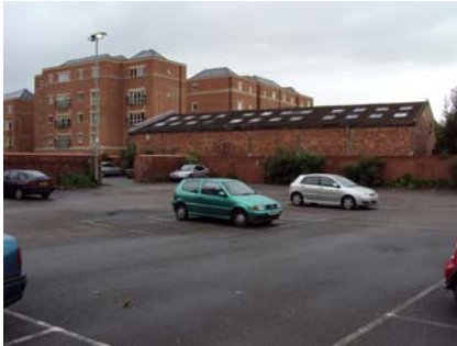
Fig 8. View of carpark to rear and adjoining residential scheme and Commercial unit
