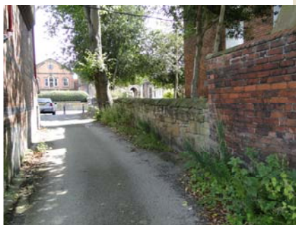
Fig 13. No 3 View of the existing dividing wall on site—To be demolished / removed
