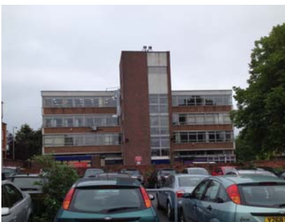
Fig 10. View of the rear of adjoining offices on Regent Street
