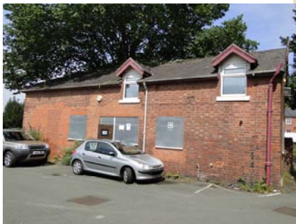
Fig 12. No 2 Former coach house is to be Demolished—To be demolished / removed
