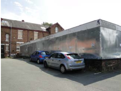
Fig 11. No 1 Portakabin accommodation to the rear of Block 1—To be demolished / removed
