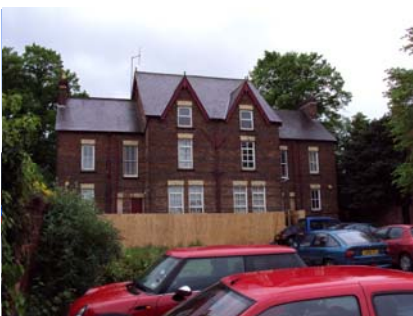
Fig 6. Rear of Block 2—previously used as Council Offices
