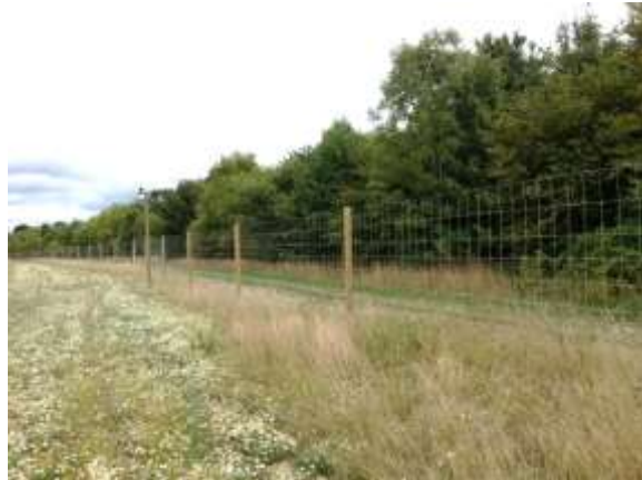
Fence at Tavells Solar Farm, Hampshire
