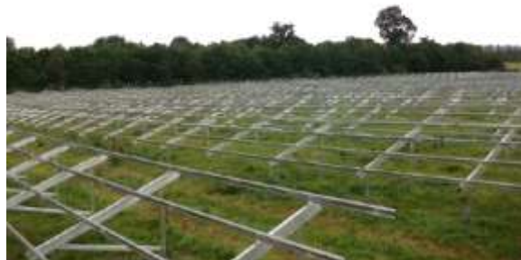
Frame structures prior to attachment of panels
