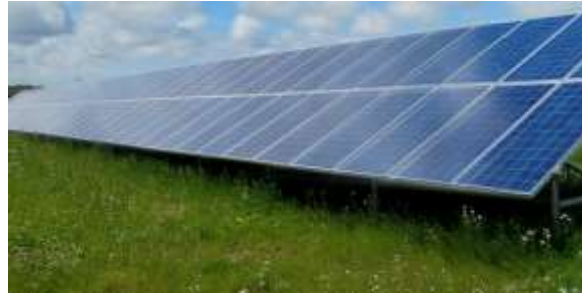
Benbole Solar Farm, Cornwall
