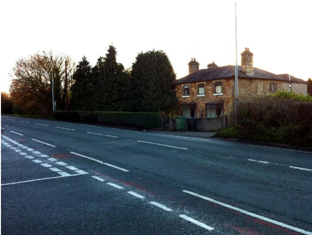
Figure 11: view of existing house and junction from junction to Crogen
