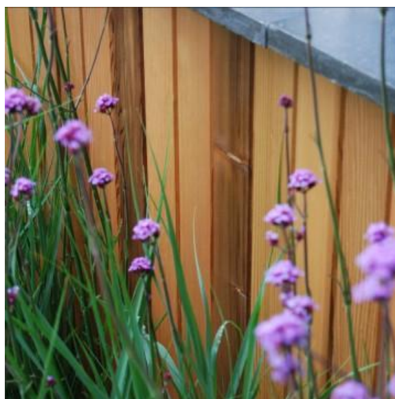
Figure 5: vertical red cedar cladding
