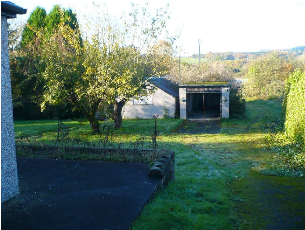
Figure 10: view of existing garages from east
