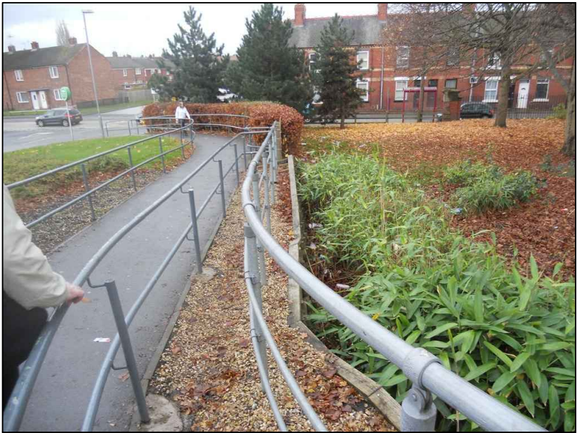
REF: D NEW PALADINE FENCING TO BE INSTALLED FROM WHERE NEW WALL FINISHES. IMAGE SHOWS POSITION WHERE A GATE WILL NEED TO BE INSTALLED AT THE END OF THE BUSH LINE. LENGTH FROM NEW WALL TO GATE: 18 METERS.
