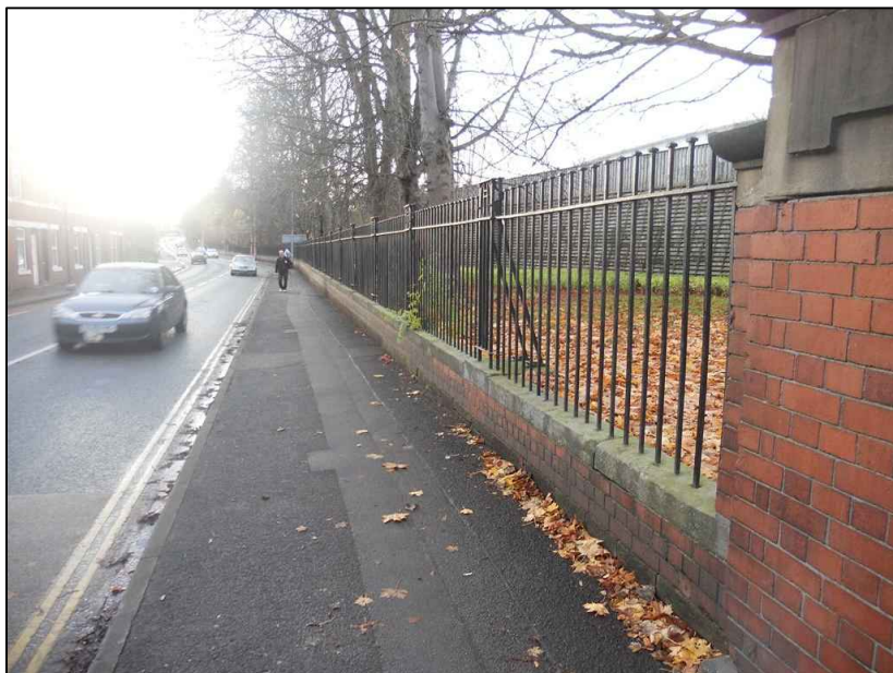
REF: A EXISTING BRICK WALL & FENCING.
