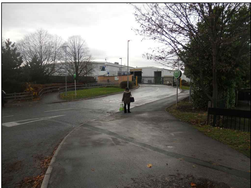
REF: G IMAGE SHOWING FULL AREA OF NEW PALADINE FENCING FROM A DISTANCE. ALSO SHOWS WHERE THE NEW WALL FINISHED AND THE NEW FENCING STARTS.
