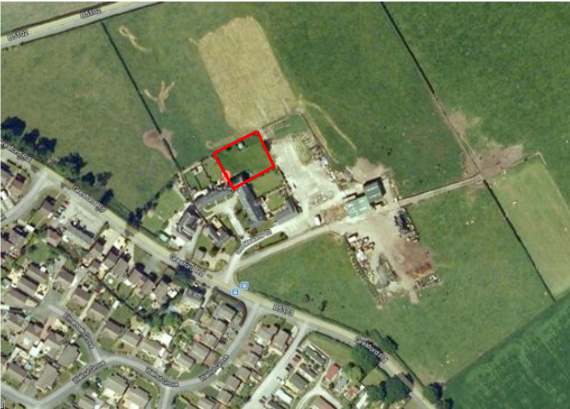
Photo 1 – aerial view of 5 The Forge: Proposal site outlined in red in centre of photo
