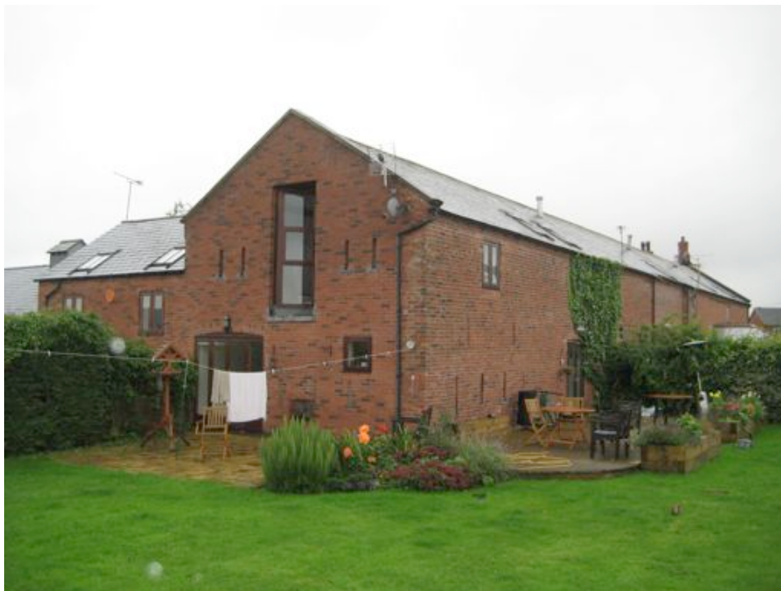
Photo 3 – Oblique view of 5 The Forge from the garden of North West and North East Elevations
