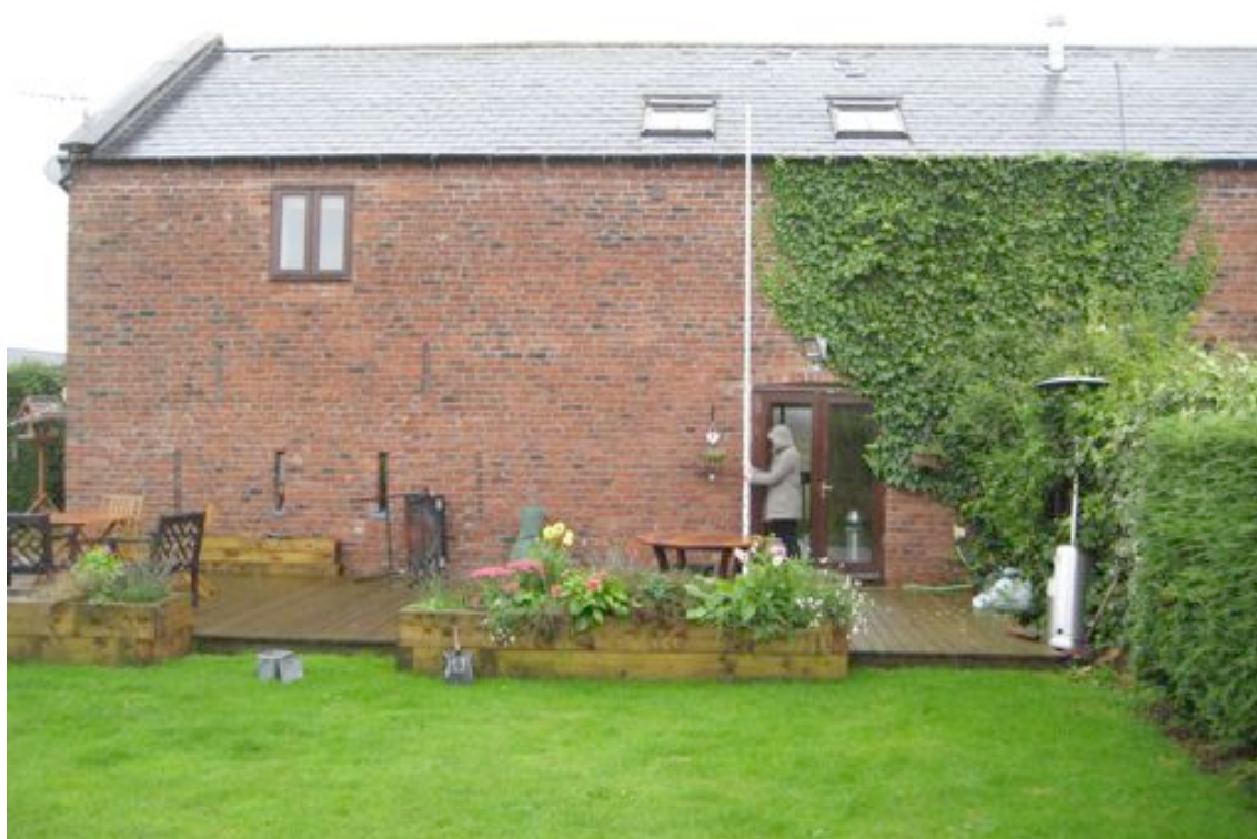
Photo 4- View of North West Elevation
