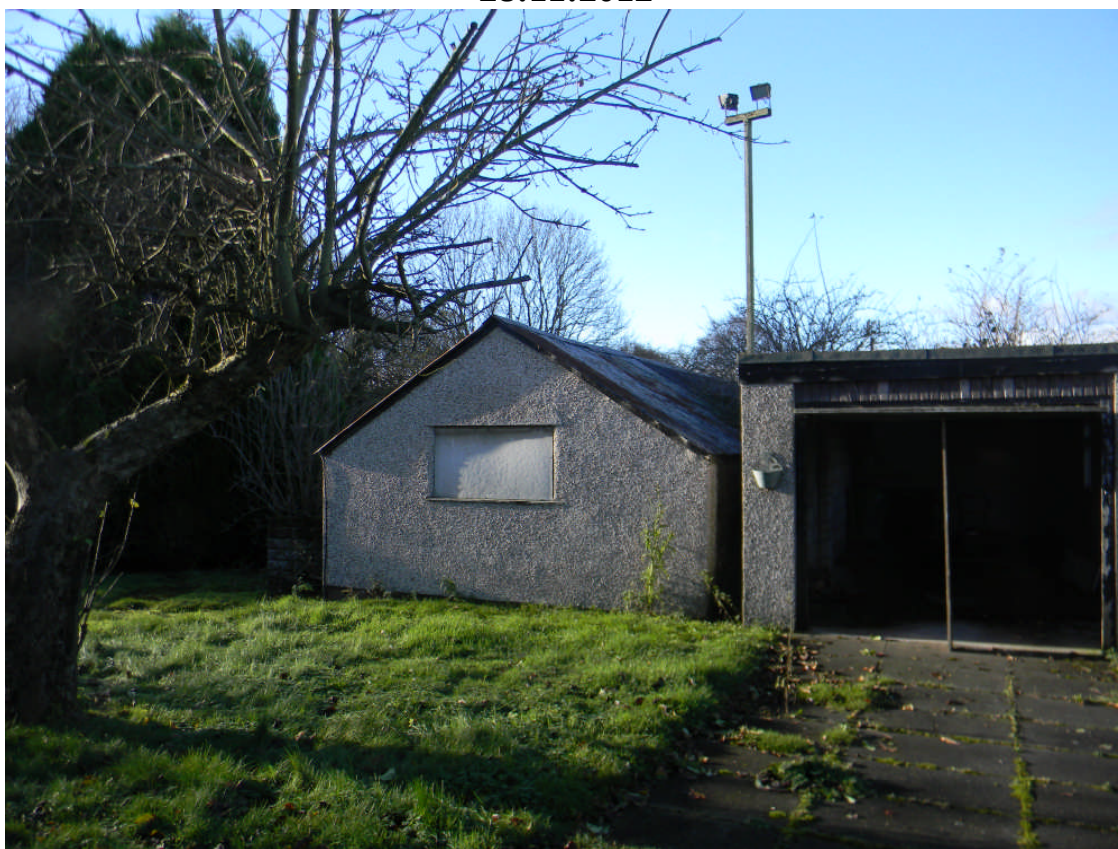
Above: The two garages proposed for demolition
