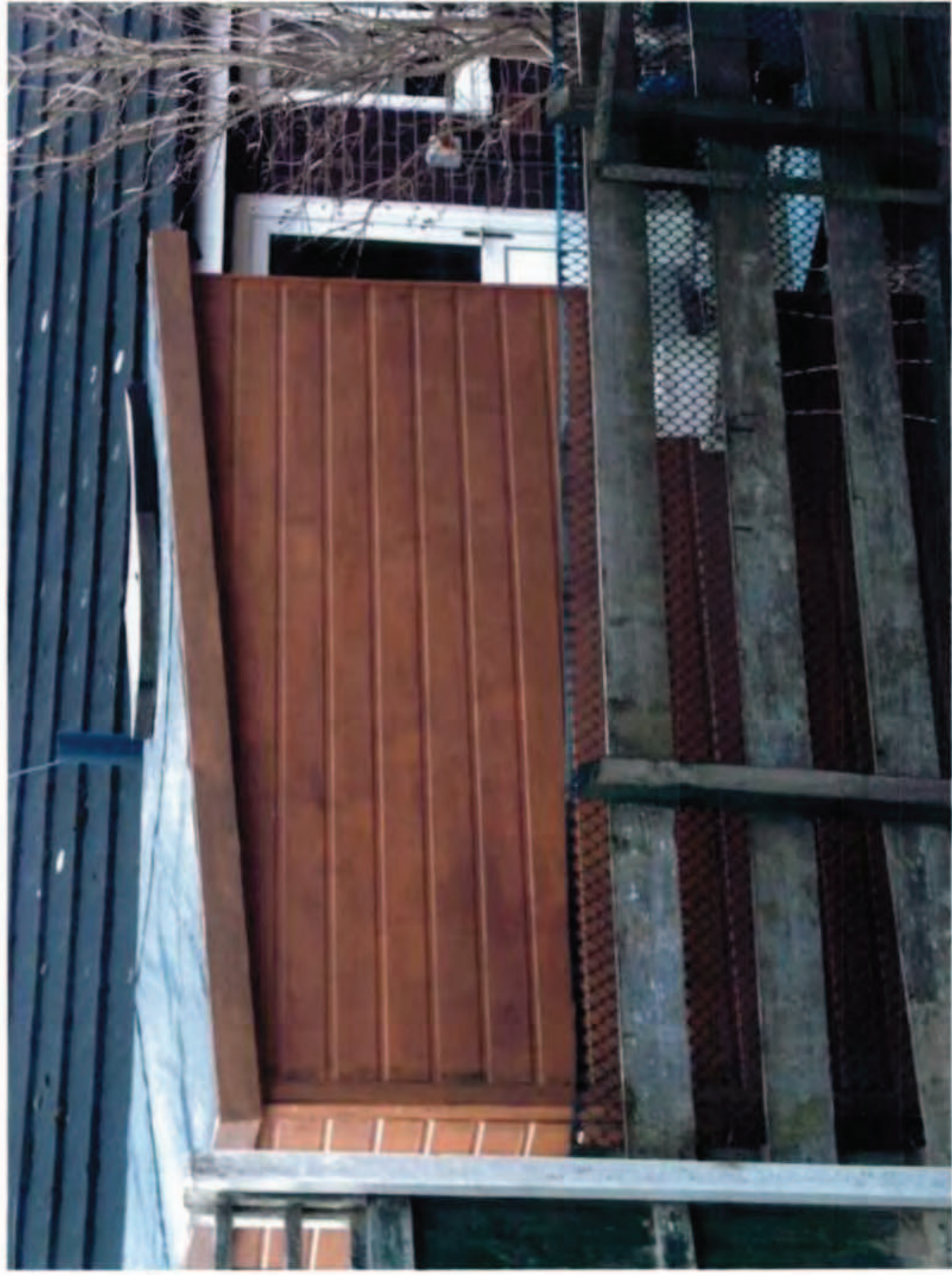
Garden Room at rear of property - Side View
