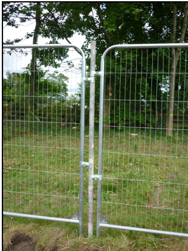
Example of Tree Protective Fencing Specification
