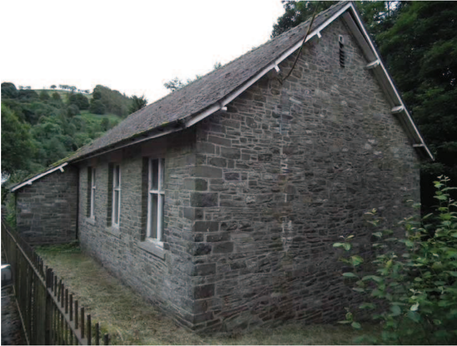
Photo 1 - Photograph of the site looking south east.
