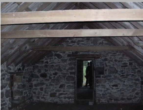
Photograph 3 – Interior of first floor of barn
