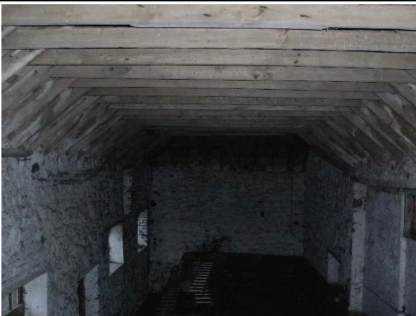
Photograph 4 – Interior of central section of barn
