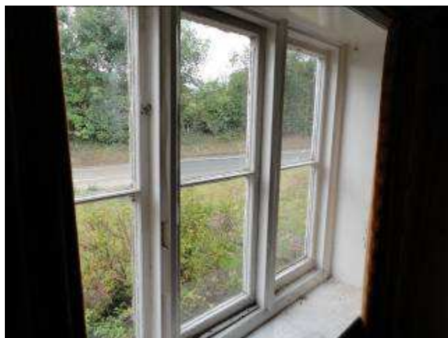
Details of typical 19 th century timber casement windows to be found throughout the property, all of which are to be repaired in-situ. Secondary glazing to be installed within the reveal of the window with mullions in-line with existing mullions and made of white powder coated aluminium.
