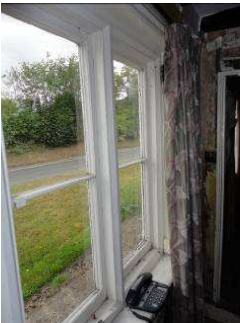
Details of typical 19 th century timber casement windows to be found throughout the property, all of which are to be repaired in-situ. Secondary glazing to be installed within the reveal of the window with mullions in-line with existing mullions and made of white powder coated aluminium.
