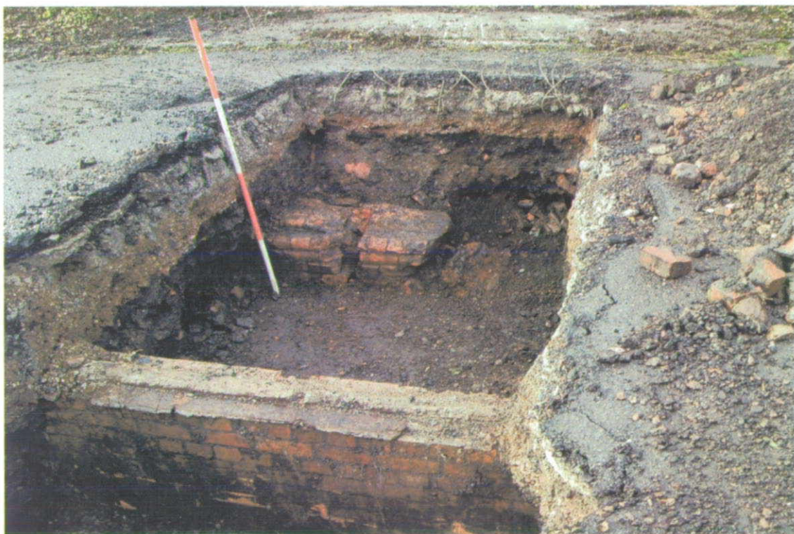
Plate 04: Tr. 2, The damaged western wall of the Compressor House. CAP Report No. 542
