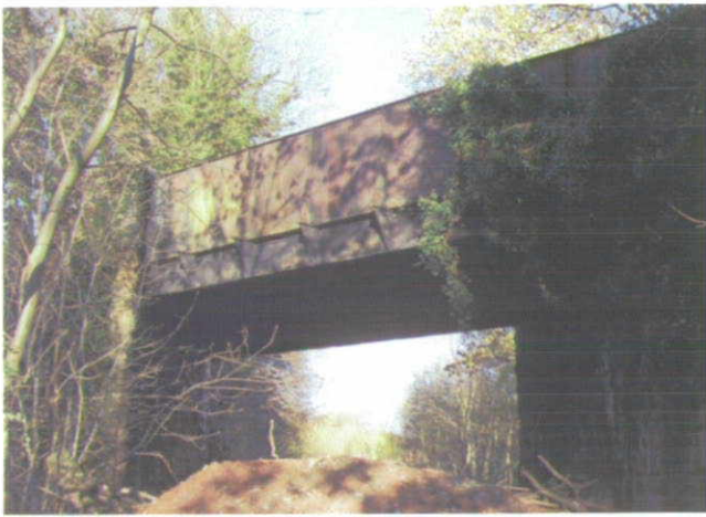
Plate 1- Bridge B1 (photograph taken from southern aspect).
