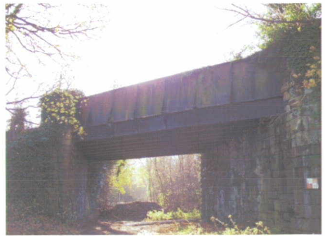
Plate 2- Bridge B1 (photograph taken from northern aspect).
