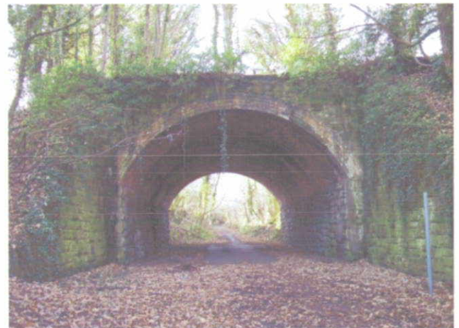
Plate 4- Bridge B2 (photograph taken from north-eastern aspect).
