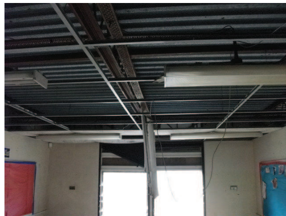
Photograph 2 – Interior of building 1
