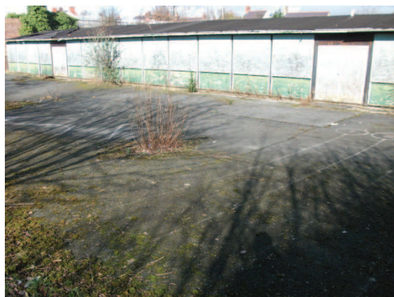
Photograph 7 – Hardstanding play area to east of site
