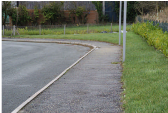
Footway along Five Crosses Dairy access road.
