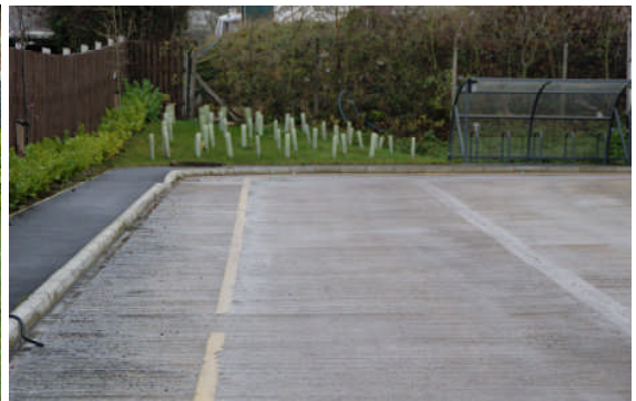
Footway, cycle route and covered cycle stand in Dairy site.
